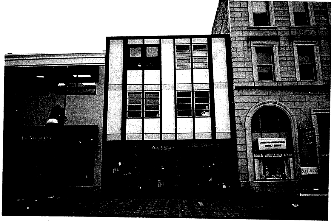
EXISTING STORE FRONT
