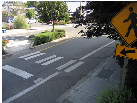
Illustration and photo of angled opening in pedestrian refuge to encourage pedestrians to view oncoming traffic.
