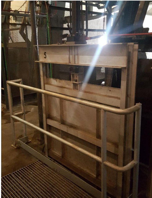
Headworks: Automatic gate that is no longer automatic
