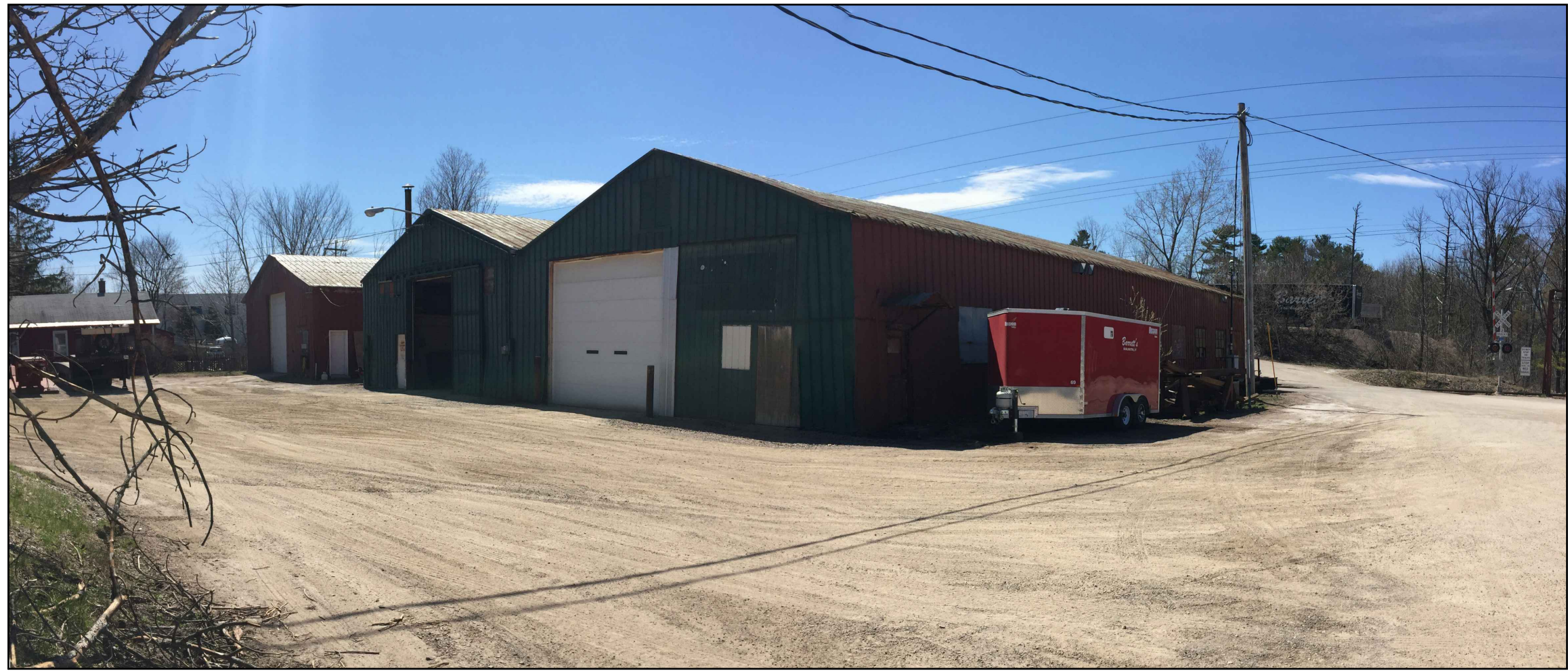
VIEW: EAST FACADE FROM BRIGGS STREET (Buildings 7&8)
