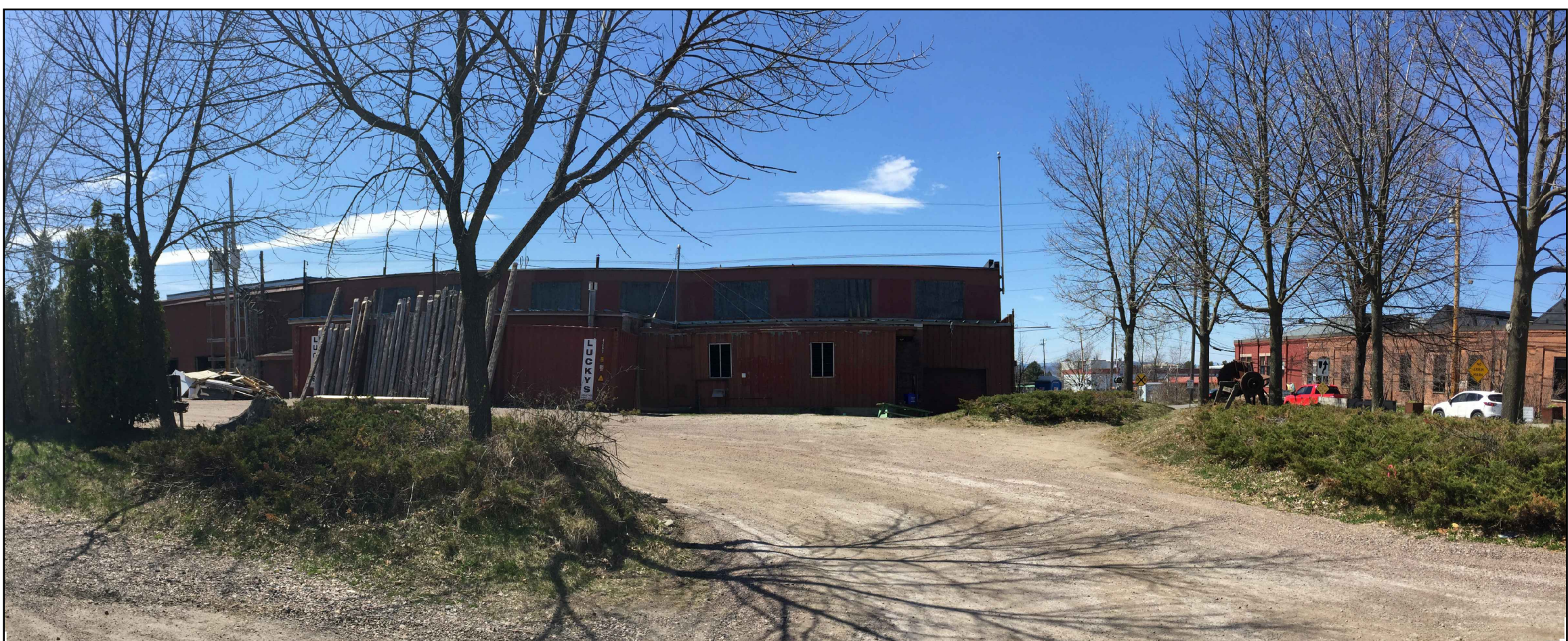
VIEW: EAST ELEVATION FROM BRIGGS STREET (Buildings 4&5)
