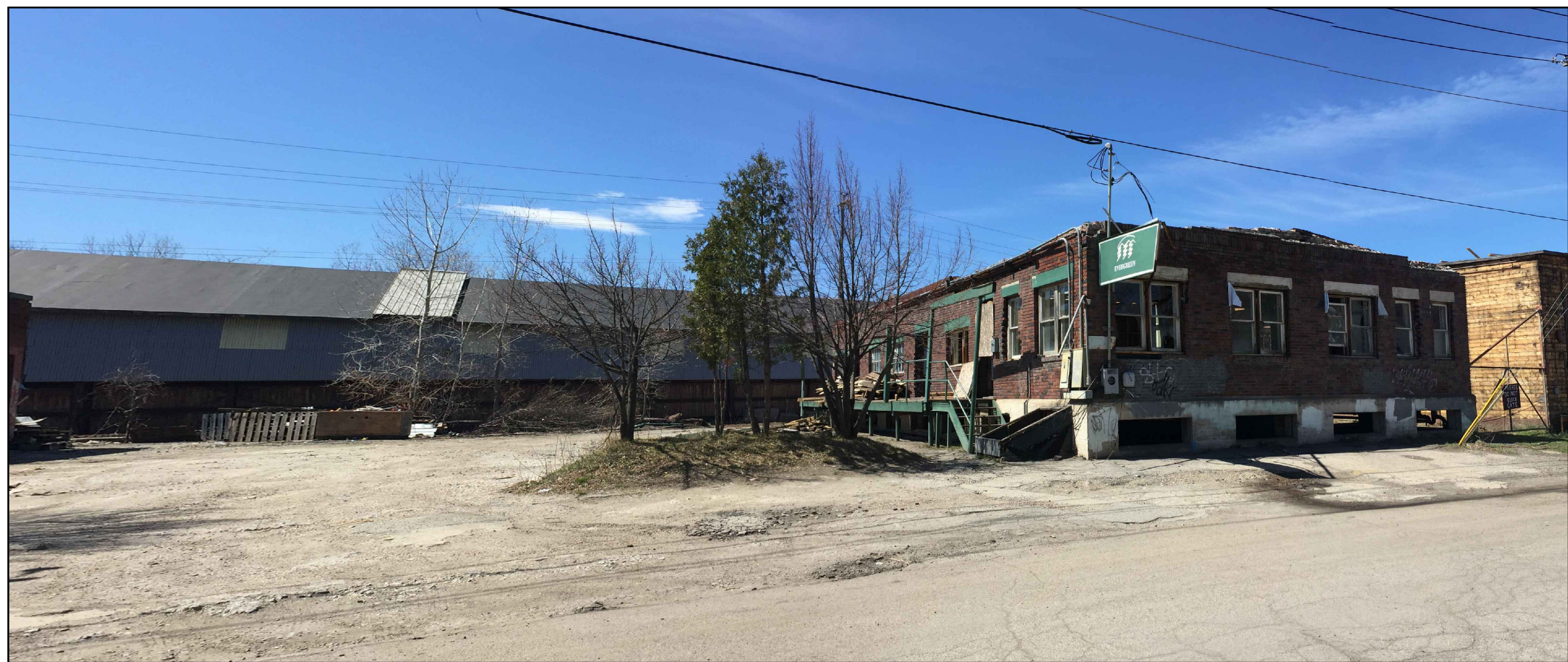
VIEW: EAST ELEVATION FROM BRIGGS STREET (Buildings 6&9)
