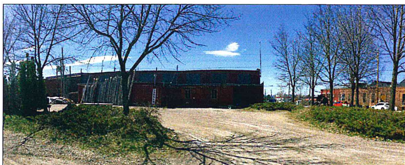
VIEW: EAST ELEVATION FROM BRIGGS STREET (Buildings 4&5)
