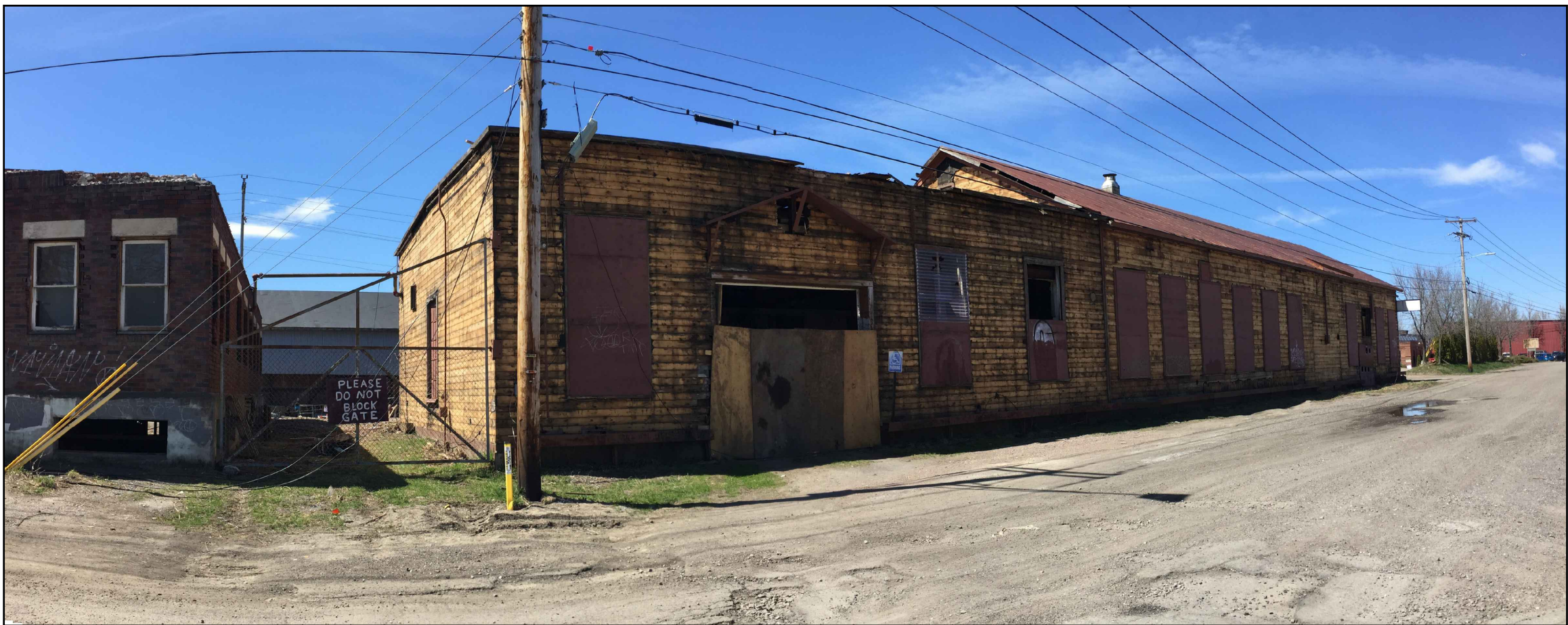
VIEW: EAST ELEVATION FROM BRIGGS STREET (Buildings 2&3)
