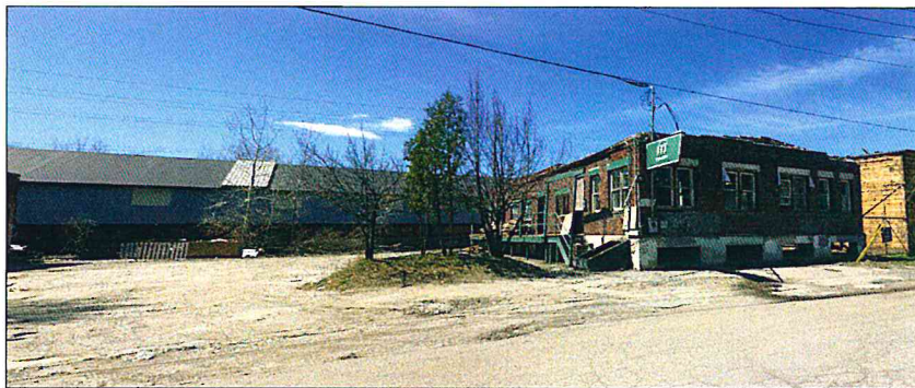
VIEW: EAST ELEVATION FROM BRIGGS STREET (Buildings 6&9)
