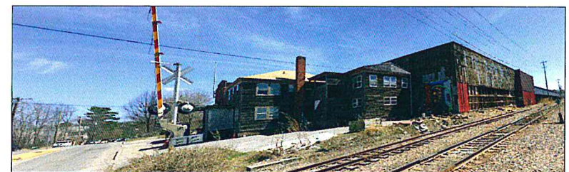
VIEW: WEST ELEVATION FROM FLYNN AVE (Buildings 1&6)
