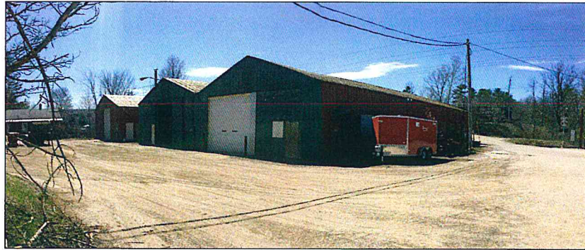
VIEW: EAST FACADE FROM BRIGGS STREET (Buildings 7&8)
