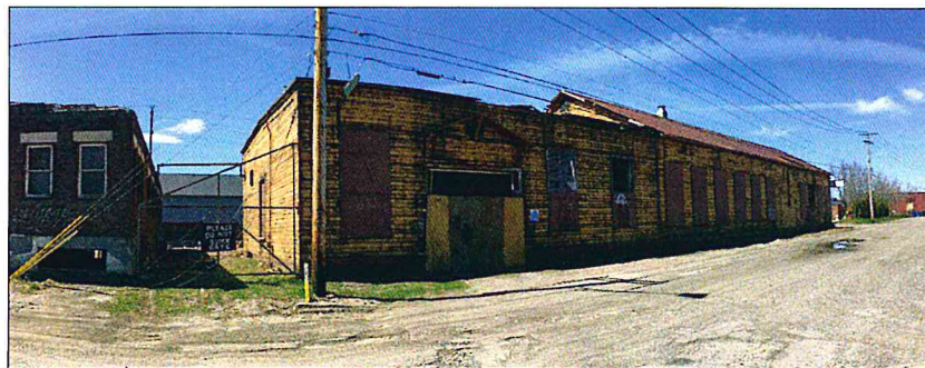
VIEW: EAST ELEVATION FROM BRIGGS STREET (Buildings 2&3)
