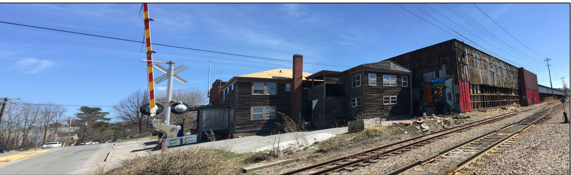
VIEW: WEST ELEVATION FROM FLYNN AVE (Buildings 1&6)
