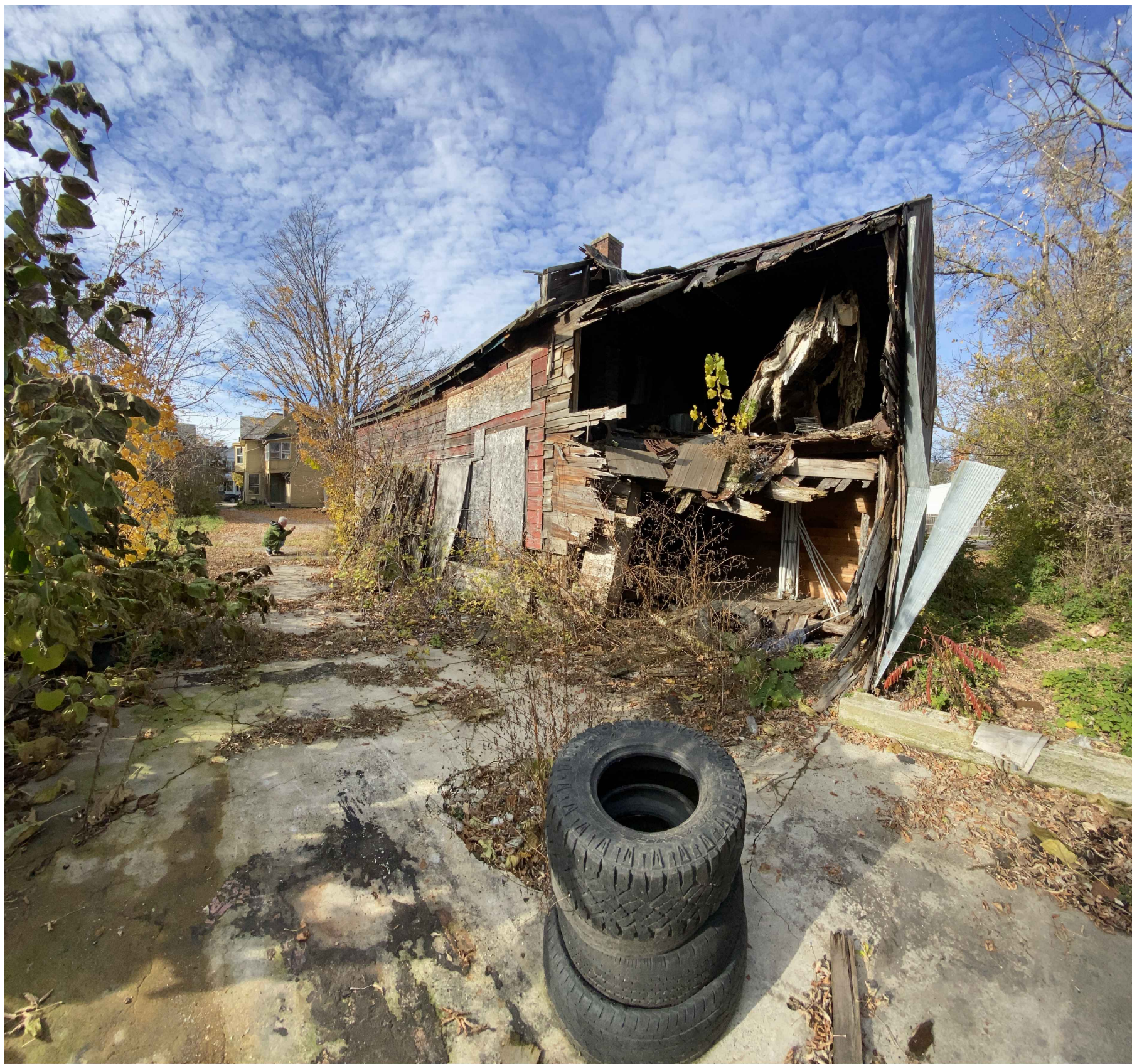
PHOTO 4 - VIEW FACING NORTHWEST
