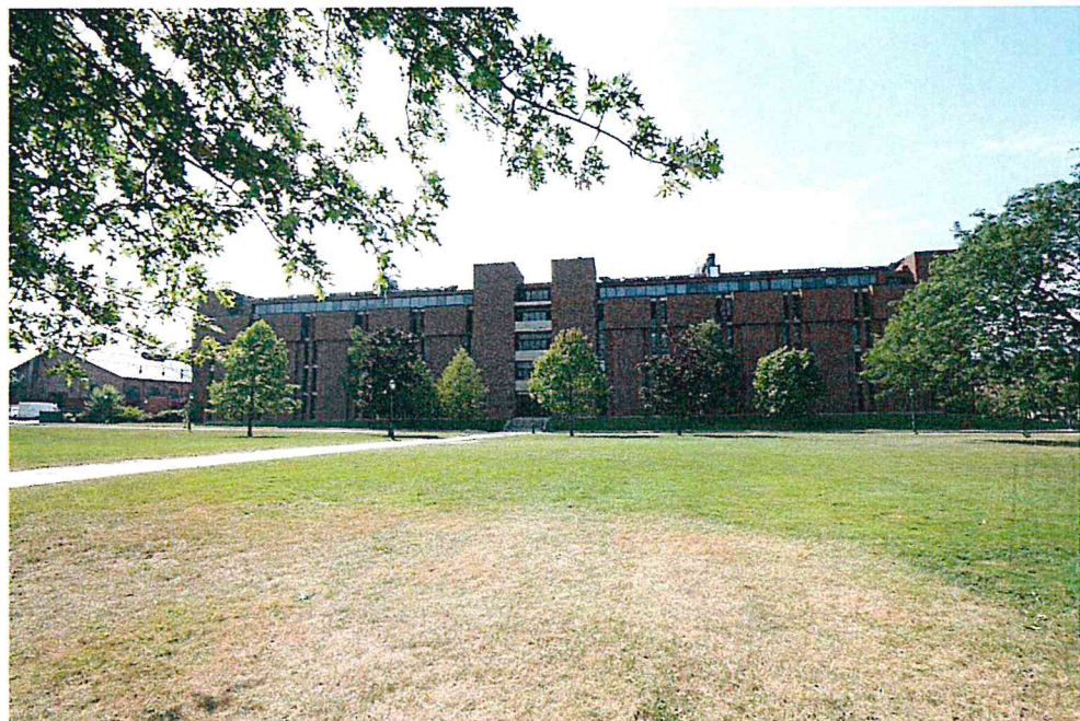
Cook, East Façade
