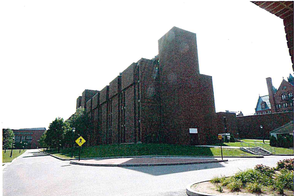
Cook, South and West Facades
