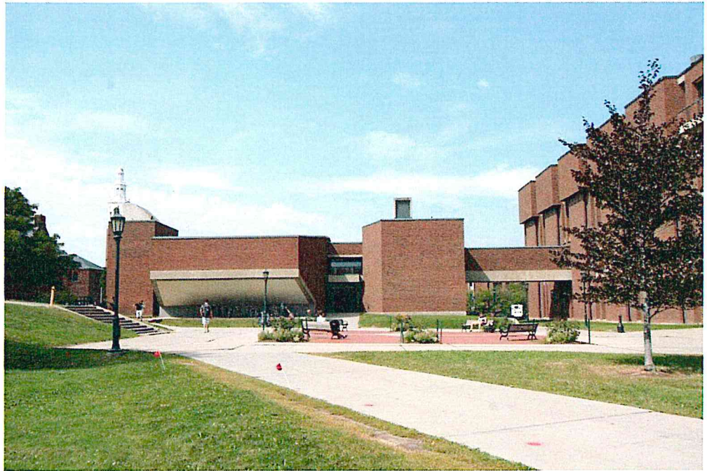
Angell, South Façade
