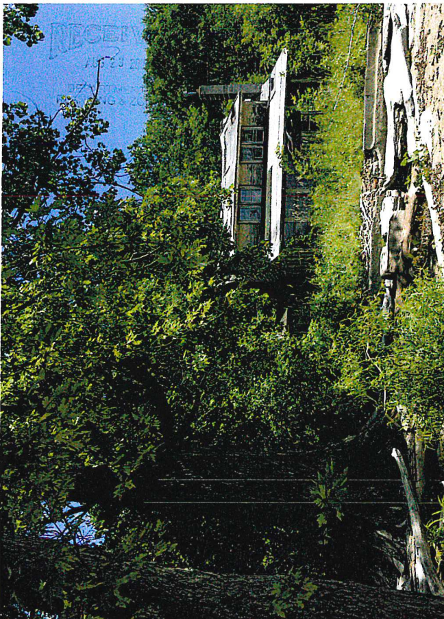
PHOTO FROM WEST LOOKING @ WEST ELEVATION OF EXISTING HOME
