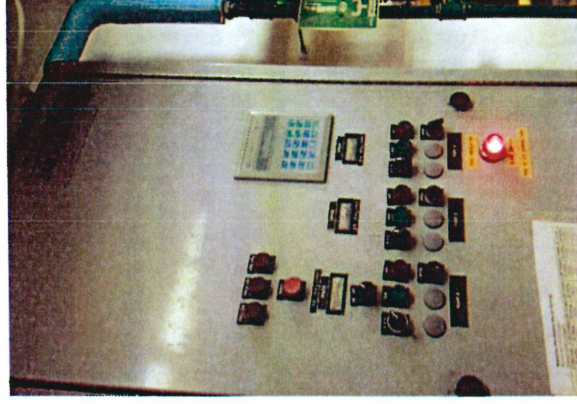
Disinfection system control panel: only one switch (hand-off-auto) works. Other control panels have obsolete parts that we cannot
