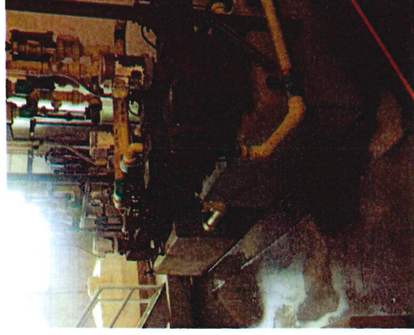
Bromine pumps: 24 years old; critical to disinfection of wet weather
