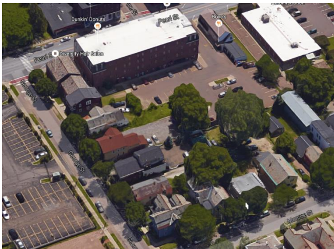
View southwest; Monroe St. at bottom right, George Street at left, Pearl Street at top.
