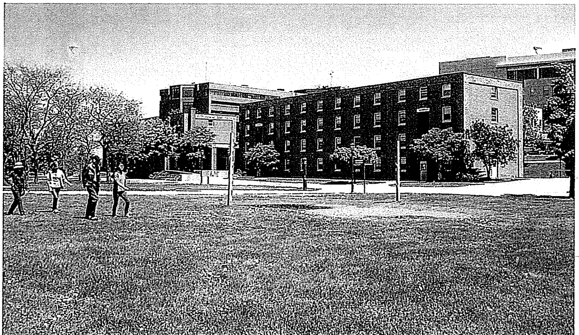
6. Additional view from the project area toward Chittenden and Buckham Halls (left to right), which will be demolished, and toward the walkways that will be reconfigured somewhat for the Green Mountain Walkway.
