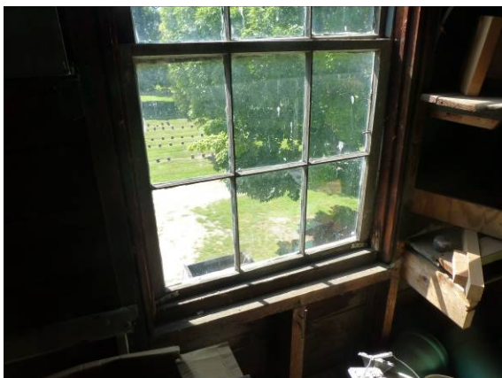
Photo #53: Maintenance building window
