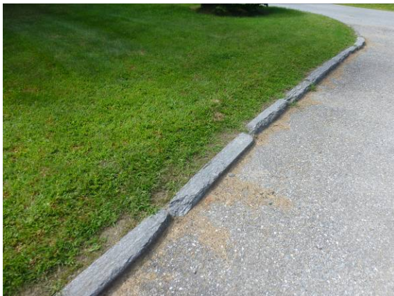
Photo #71: Curbing detail
