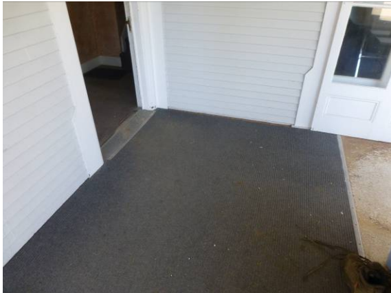
Photo #25: Porch flooring detail
