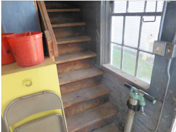
Photo #49: Maintenance building stairs
