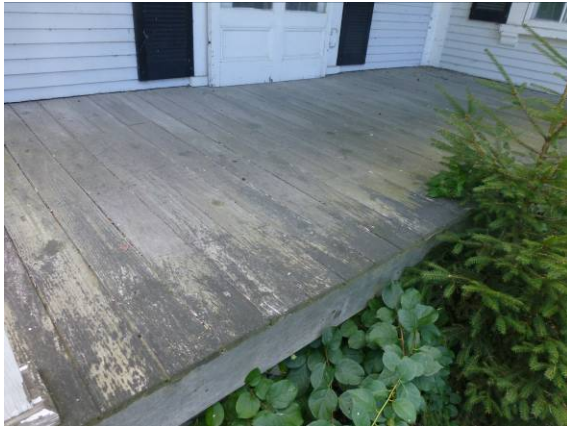
Photo #13: Cemetery building porch
