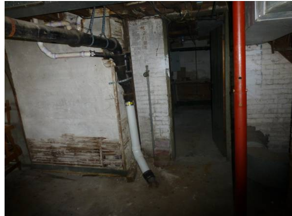
Photo #32: Basement area
