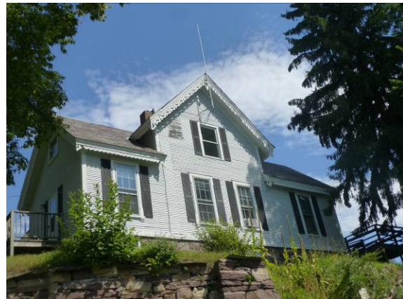
Photo #4: West elevation of cemetery building
