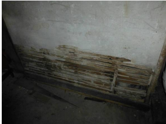
Photo #31: Wall detail
