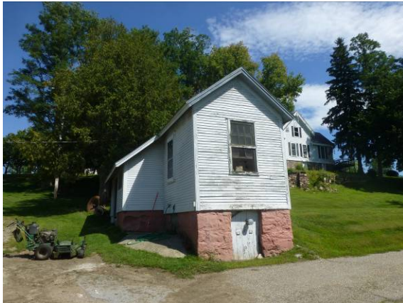
Photo #55: Break house exterior elevation
