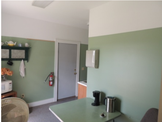
Photo #91: Fire extinguisher
