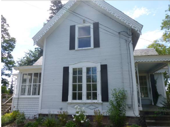
Photo #1: East elevation of cemetery building
