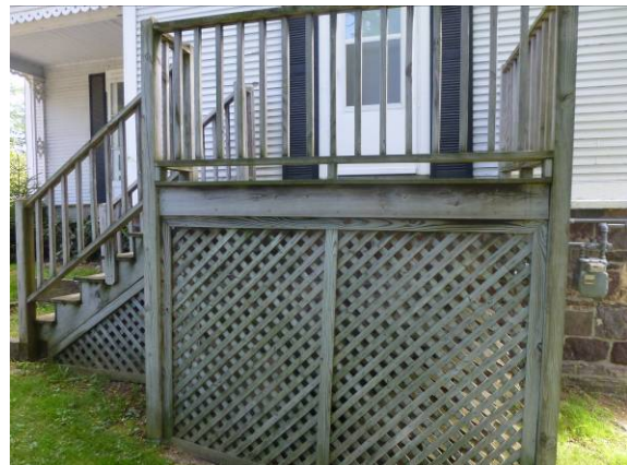
Photo #10: Cemetery building stairs
