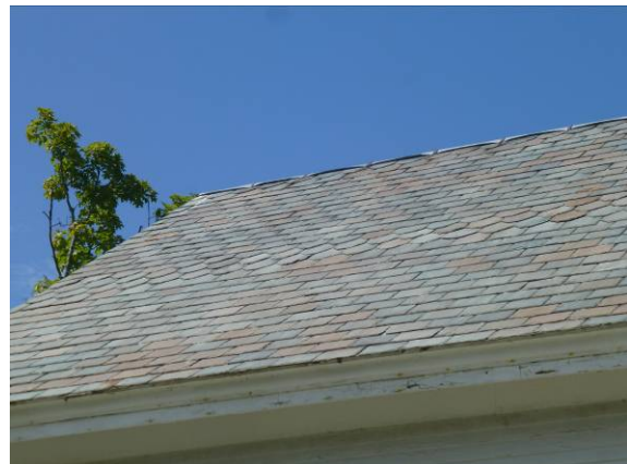
Photo #46: Maintenance building roof
