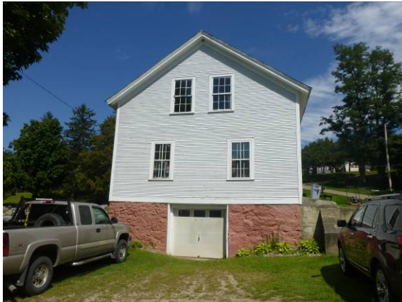
Photo #43: Maintenance building exterior elevation
