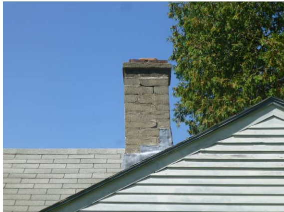
Photo #61: Break house chimney
