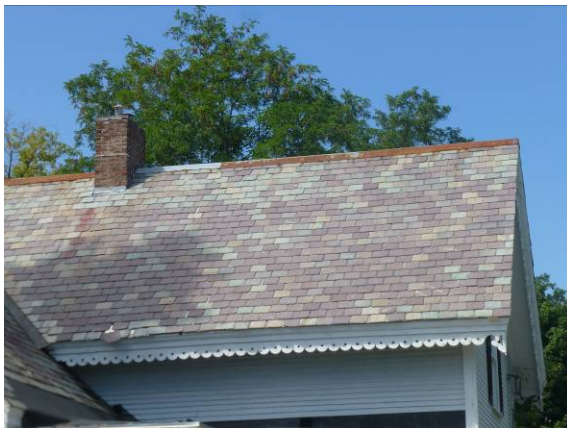
Photo #5: Cemetery building roof
