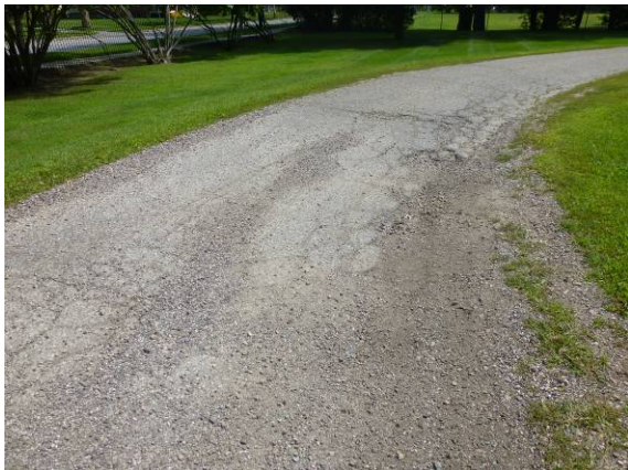
Photo #69: Drive aisle
