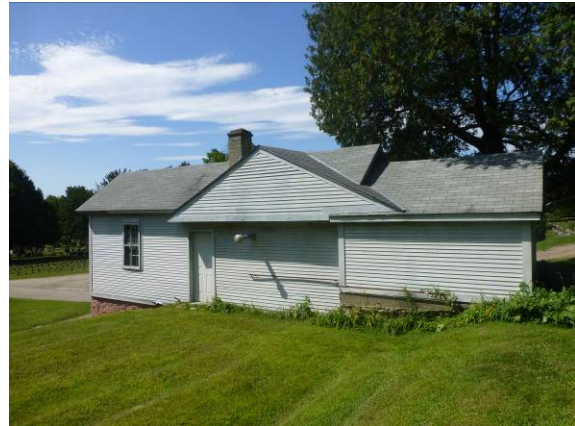
Photo #56: Break house exterior elevation
