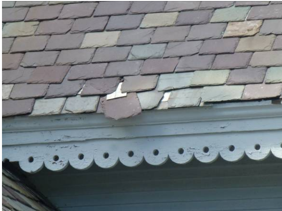
Photo #7: Cemetery building roof detail
