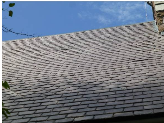
Photo #39: Chapel slate roof
