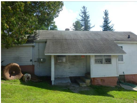
Photo #57: Break house exterior elevation
