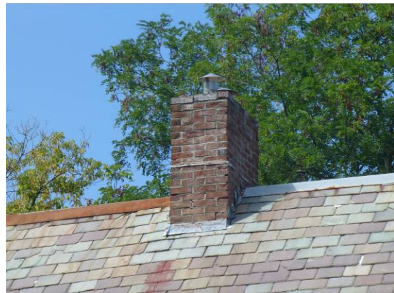
Photo #6: Cemetery building chimney
