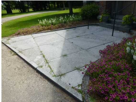
Photo #37: Chapel paving detail
