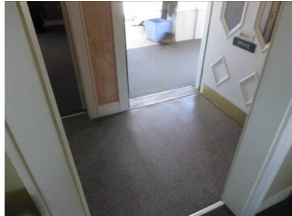
Photo #26: Entrance flooring detail
