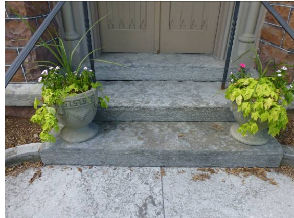
Photo #38: Chapel stair detail
