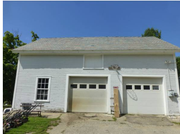
Photo #44: Maintenance building exterior elevation
