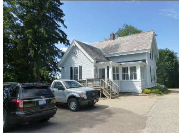
Photo #2: South elevation of cemetery building
