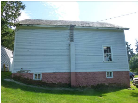
Photo #45: Maintenance building exterior elevation
