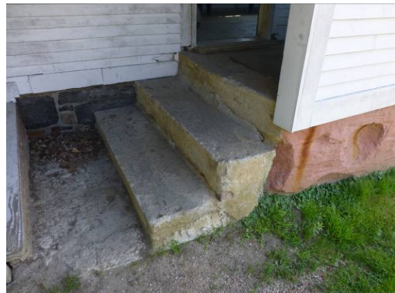
Photo #58: Break house exterior stairs
