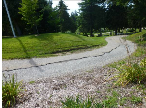
Photo #68: Drive aisle
