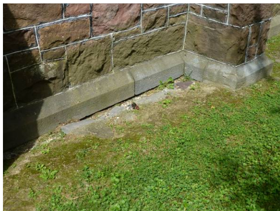
Photo #41: Chapel foundation detail
