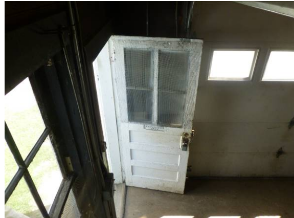
Photo #50: Maintenance building door
