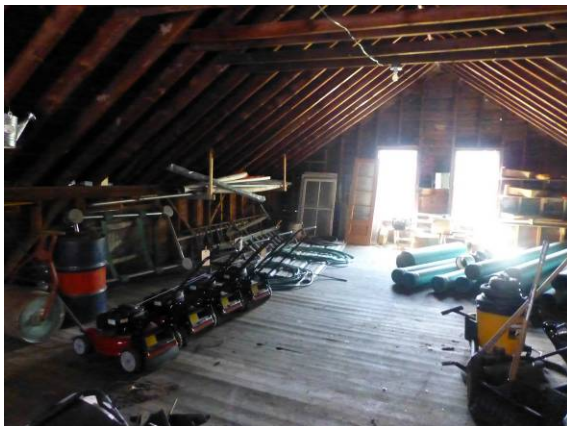
Photo #51: Maintenance building interior attic space
