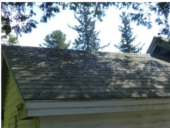
Photo #59: Break house roof
