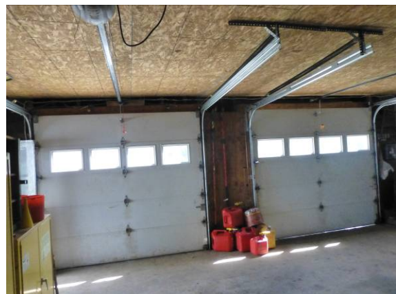
Photo #48: Maintenance building overhead doors
