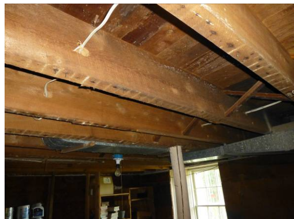
Photo #30: Floor structure
