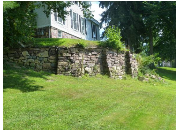
Photo #76: Retaining wall
