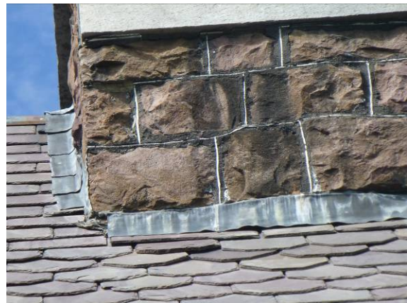
Photo #40: Chapel chimney detail
