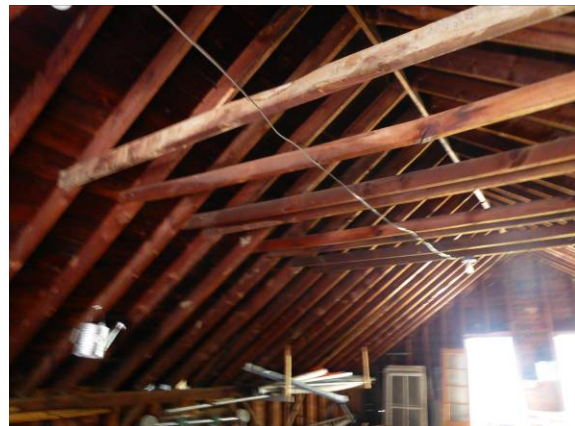
Photo #52: Maintenance building structure
