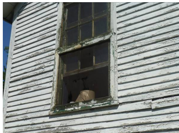
Photo #60: Break house window
