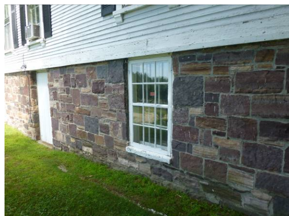
Photo #12: Cemetery building foundation
