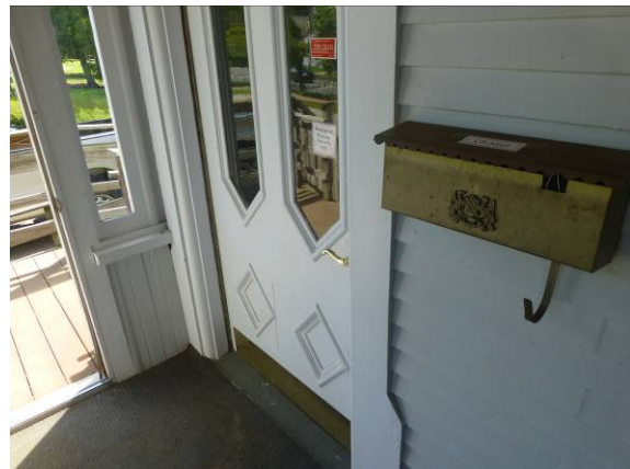
Photo #16: Entrance door
