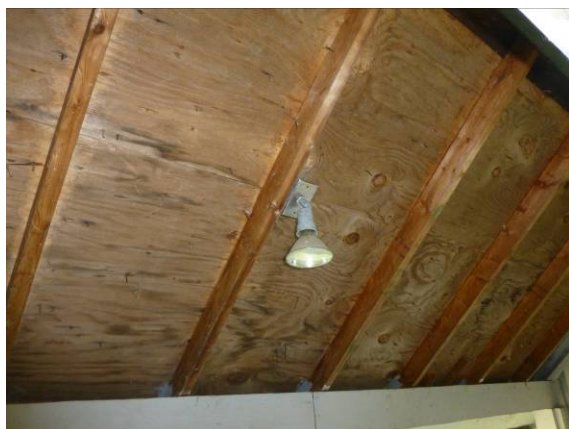
Photo #65: Break house roof structure
