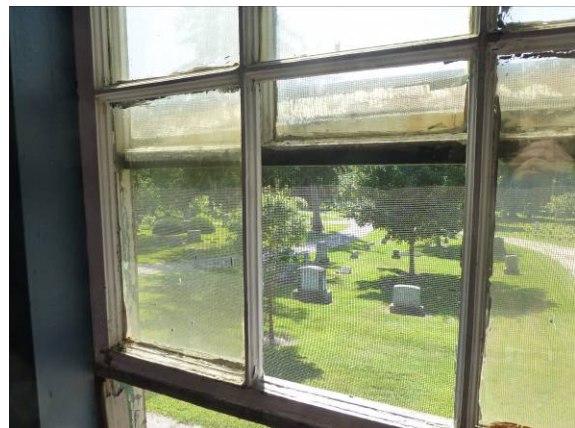
Photo #64: Break house window detail
