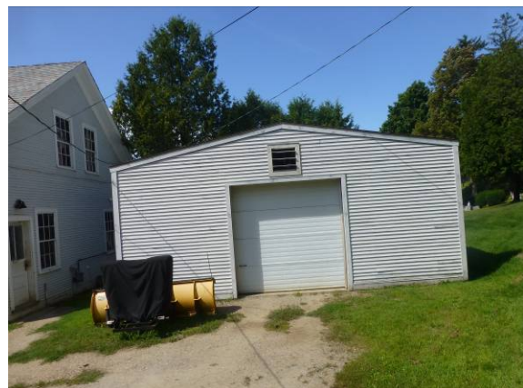
Photo #54: Storage building
