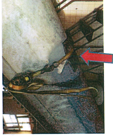
Corroded metal components: Full of bandaids and patches or not easily repairable.
