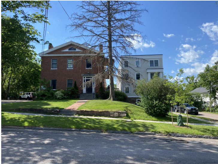
VIEW TO SOUTH FROM COLLEGE STREET
