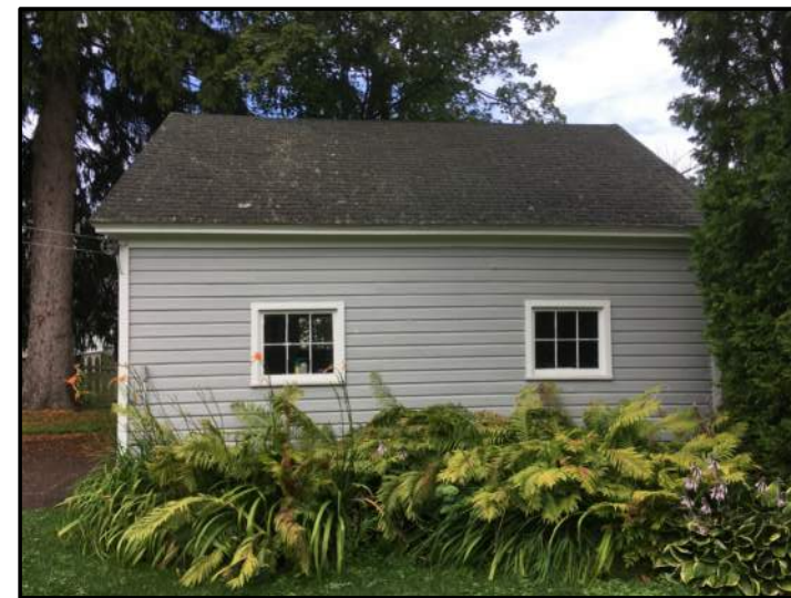
EXISTING GARAGE - EAST FACADE
