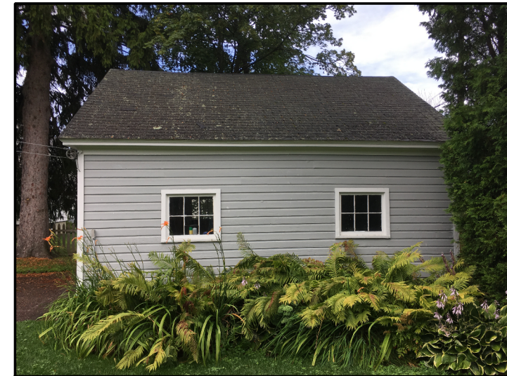
EXISTING GARAGE - EAST FACADE
