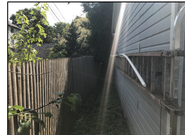
EXISTING GARAGE - NORTH (REAR) SETBACK
