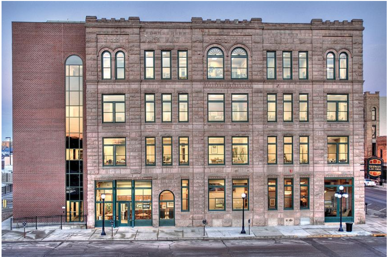
“Figure 27a. The compatible addition is set back and does not compete with the historic building. Photo: Chadd Gossmann, Aurora Photography, LLC” Preservation Brief 14: New Exterior Additions to Historic Buildings: Preservation Concerns (nps.gov) . Please note that the new exterior addition has fenestrations that echo the aesthetic rhythm of the historic structure in a more creative way – the new windows are larger, allowing more light.
