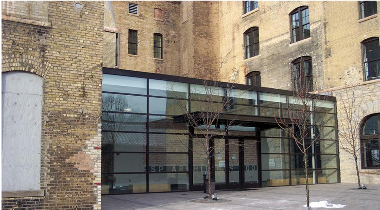
“Figure 14. This glass addition was erected at the back of an 1895 former brewery during rehabilitation to provide another entrance. The addition is compatible with the plain character of this secondary elevation.” Preservation Brief 14: New Exterior Additions to Historic Buildings: Preservation Concerns (nps.gov) Note that on a rear elevation, the standard for assessing compatibility is given much more room for interpretation – in this case, an all glass enclosure is still seen as “plain” in total even though the fenestrations do not match the existing historic fenestrations. The addition is assessed as a whole.
