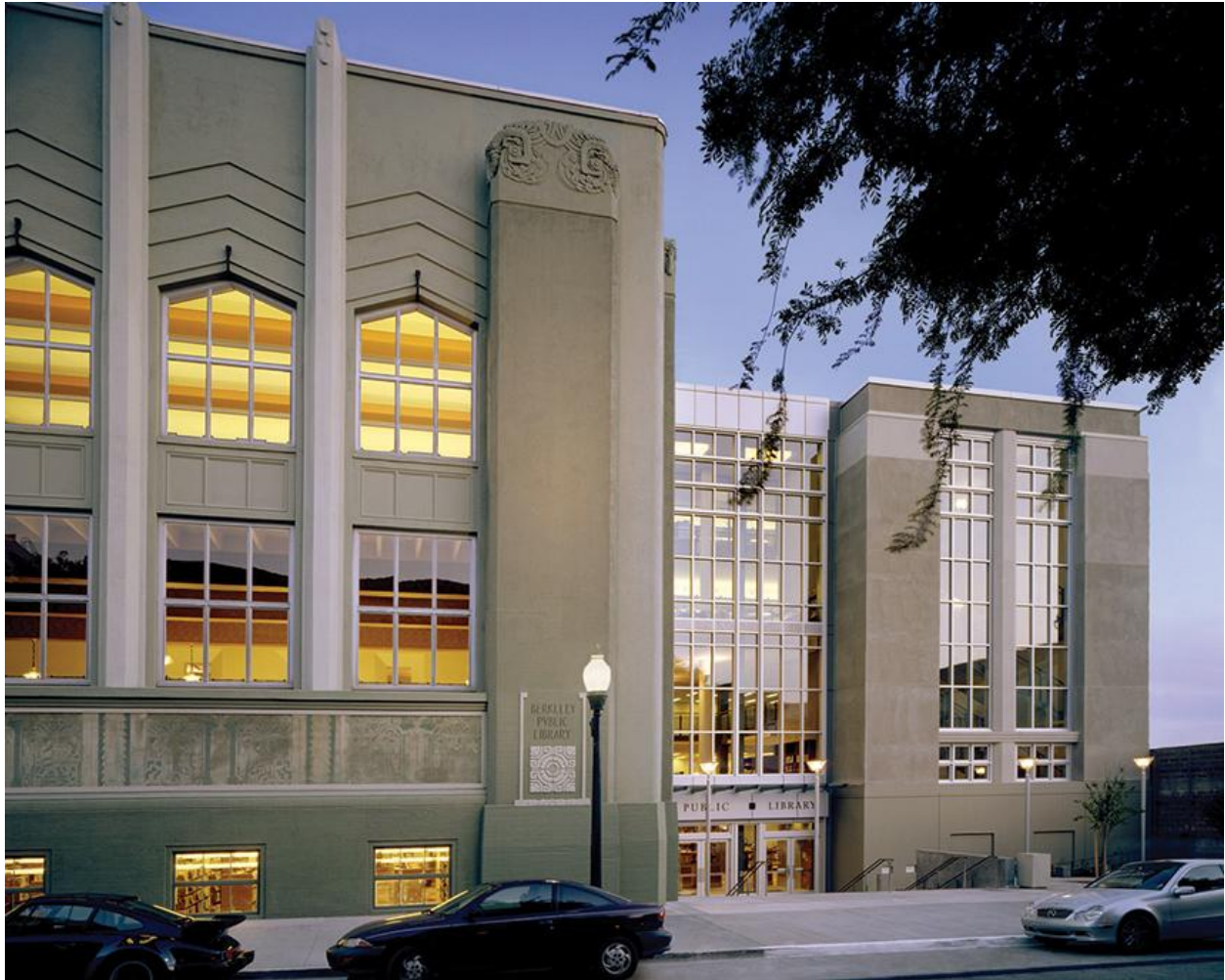
Figure 1. The addition to the right with its connecting hyphen is compatible with the Collegiate Gothic-style library. The addition is set back from the front of the library and uses the same materials and a simplified design that references, but does not copy, the historic building. Photo: David Wakely Photography. Preservation Brief 14: New Exterior Additions to Historic Buildings: Preservation Concerns (nps.gov) Note that fenestrations borrow ratios from other design elements while favoring the ability to bring in maximum natural light.
