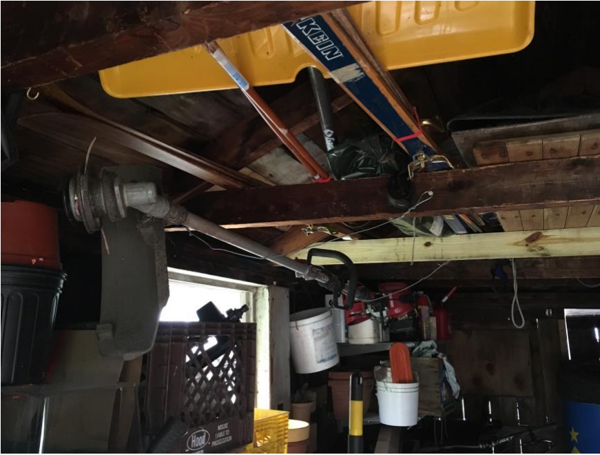
Secured existing ceiling joists and added additional joists in fall 2017
