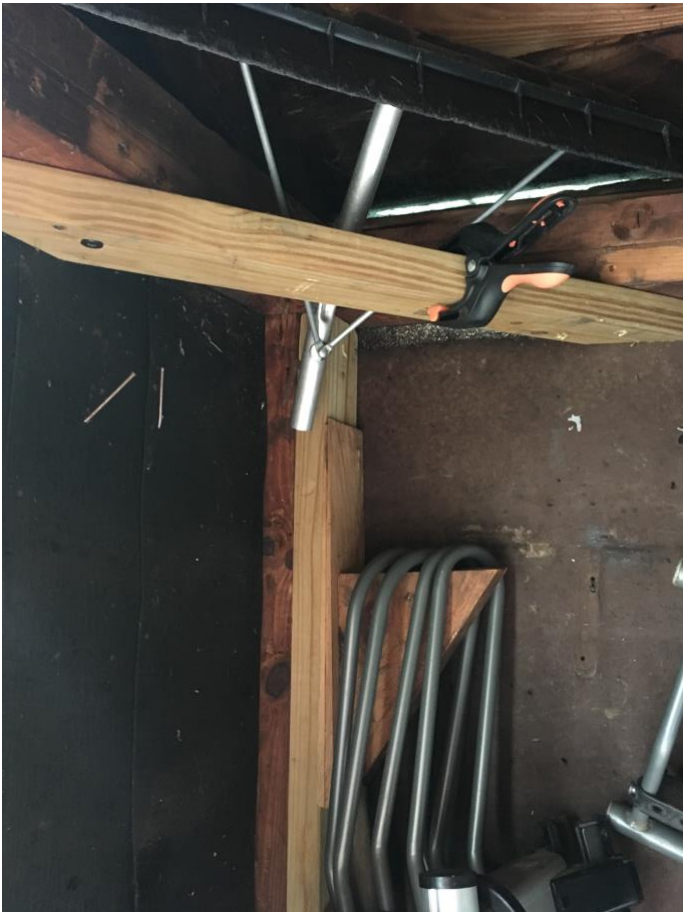
Reinforced corners in fall 2017
