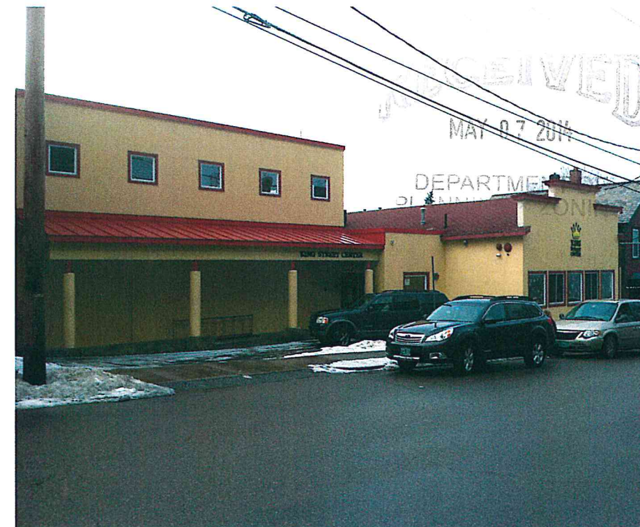
Existing King Street Center (With Existing Signs Removed during Demolition)
