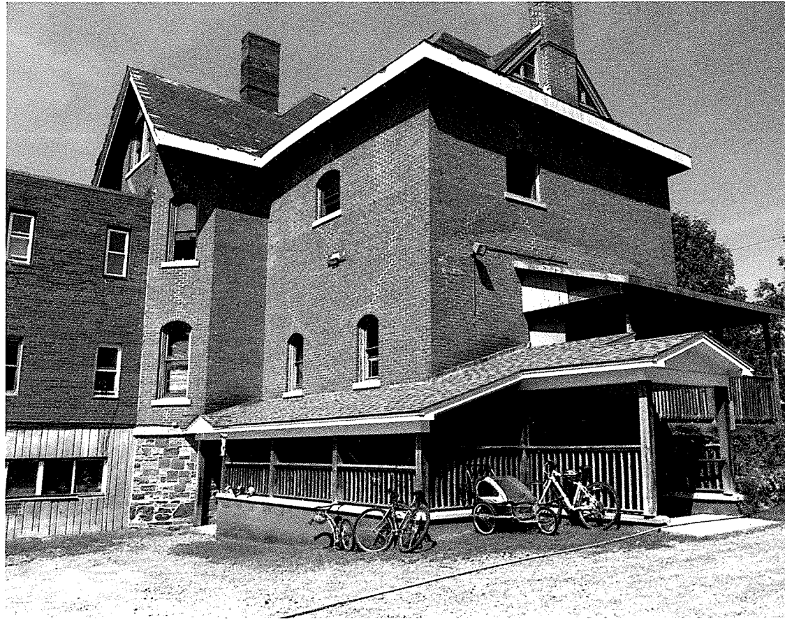
Current Side Entrance
