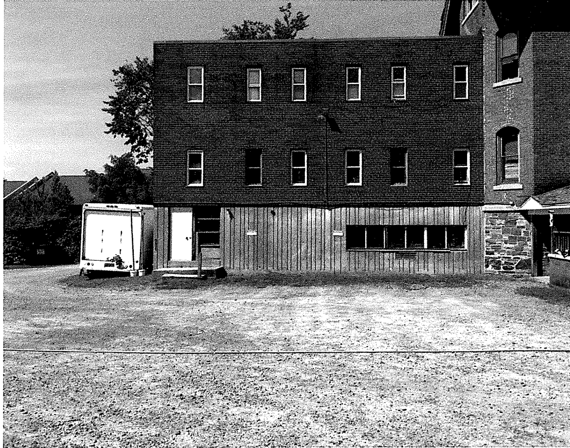
Current Rear of Building – South Elevation
