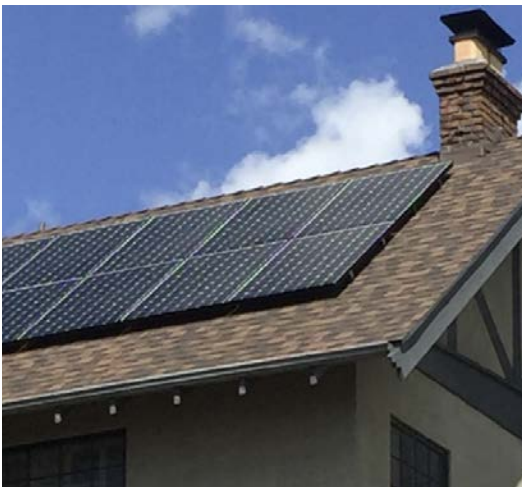
Solar array mounted on an historic home.
