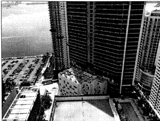
Looking up at the 13-level 480-car Robotic Valet™ garage at the Brickellhouse condominium in Miami, Florida. (Woody Nash, Boomerang Systems, Inc. Photo: Michael J. Paddon)
