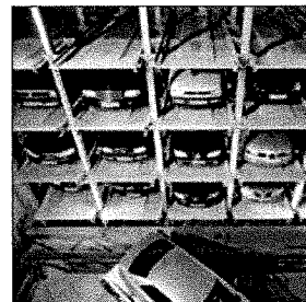
Summit Grand Parc (Courtesy of Space Saver Parking Company and Mid-American Elevator Company)
