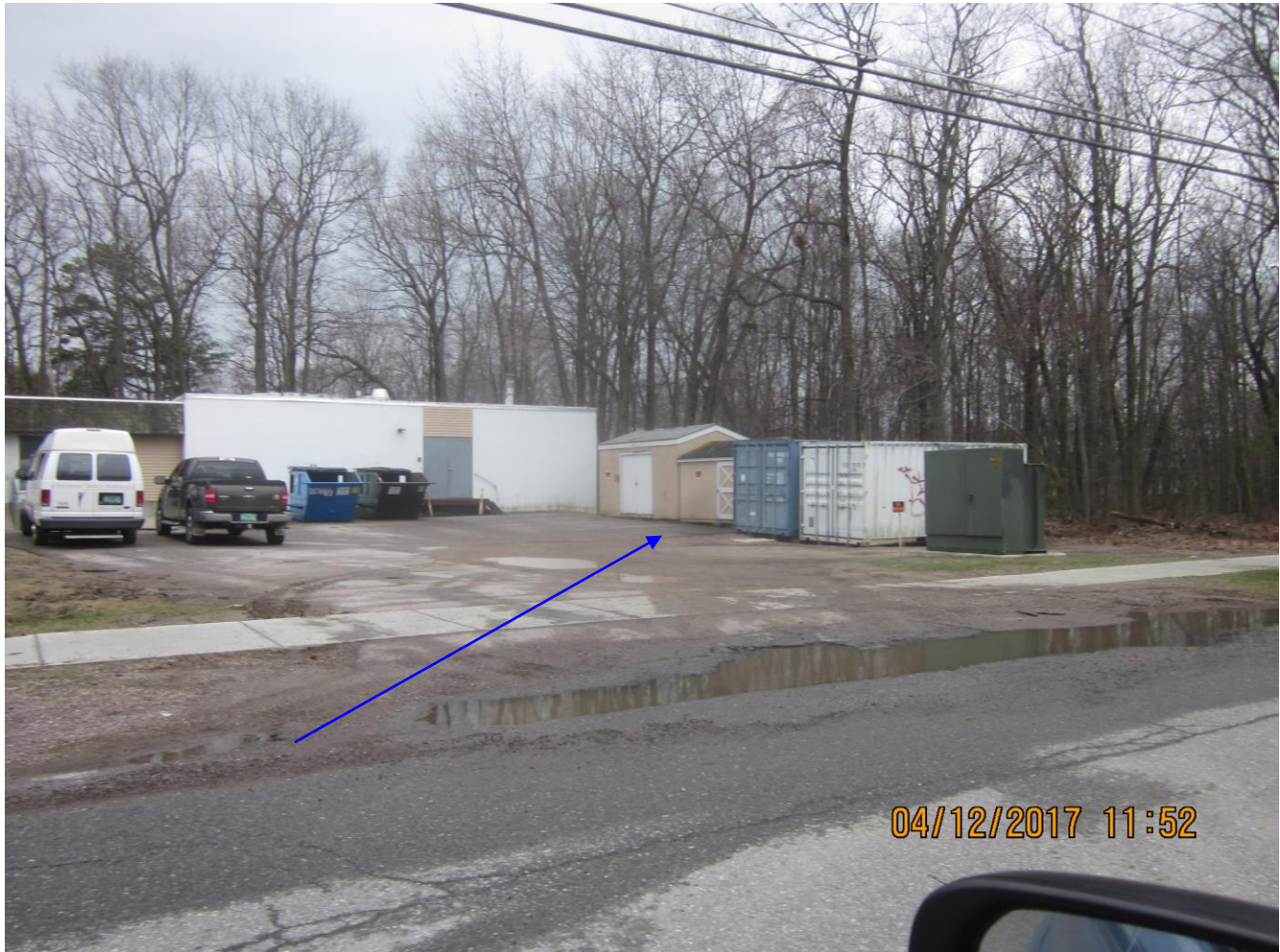
North of loading dock. Two sheds (one with hazardous waste) and two storage containers do not have zoning approval.
