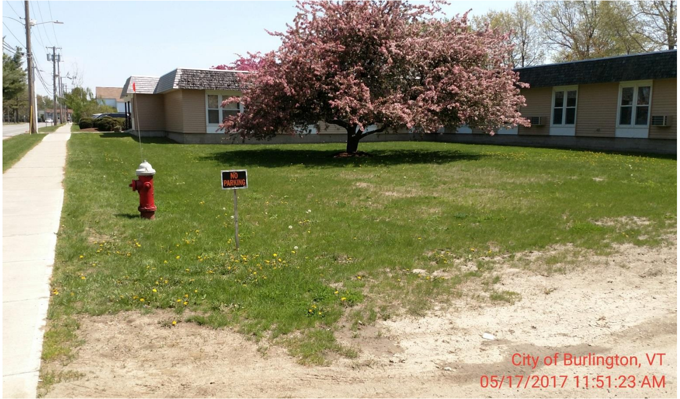
Area E: At the corner of Driveway E. Unpermitted parking has damaged the lawn and must be restored.
