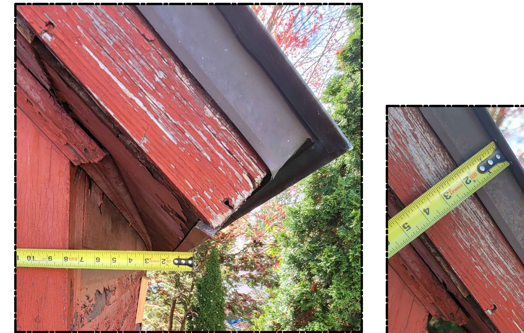
② Typical Eave Detail, Existing
