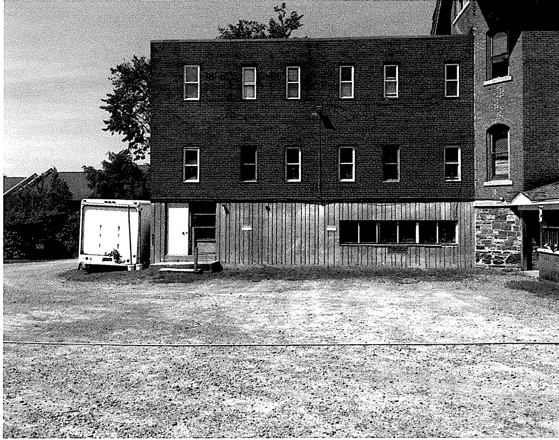
Current Rear of Building – South Elevation
