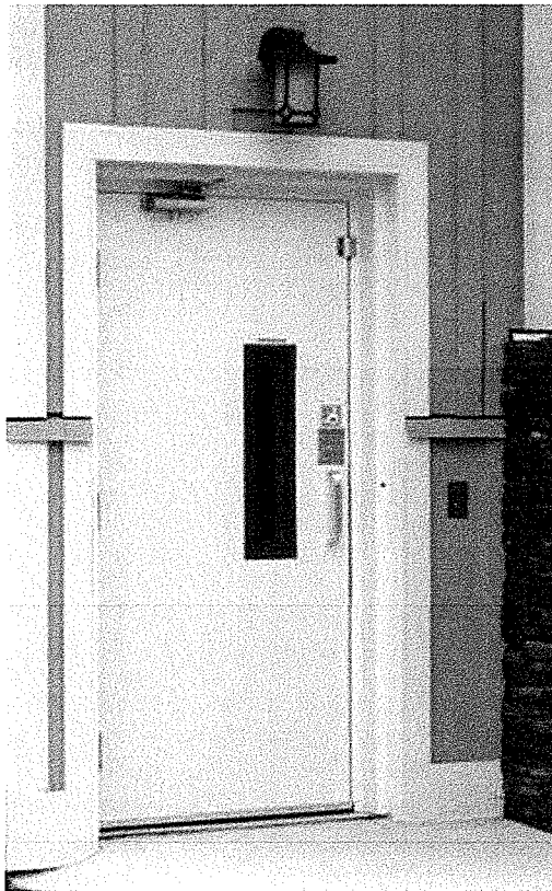
Vertical platform lift with a full height cab
