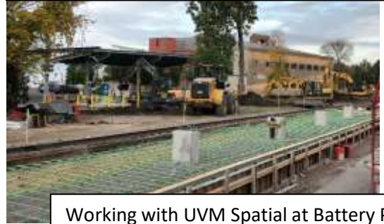
Greenway and track realignment project
