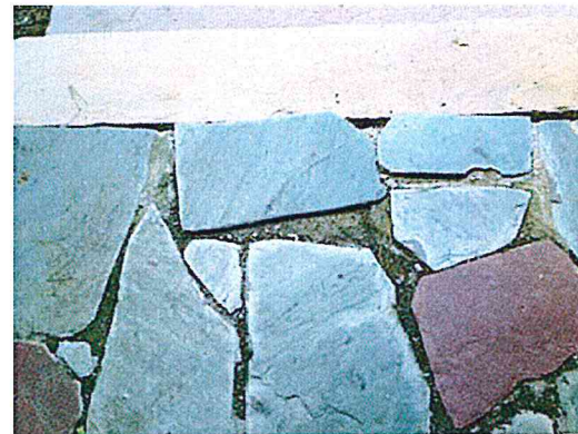
Current condition of porch floor slate
