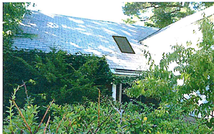
Approximate location of proposed skylight
