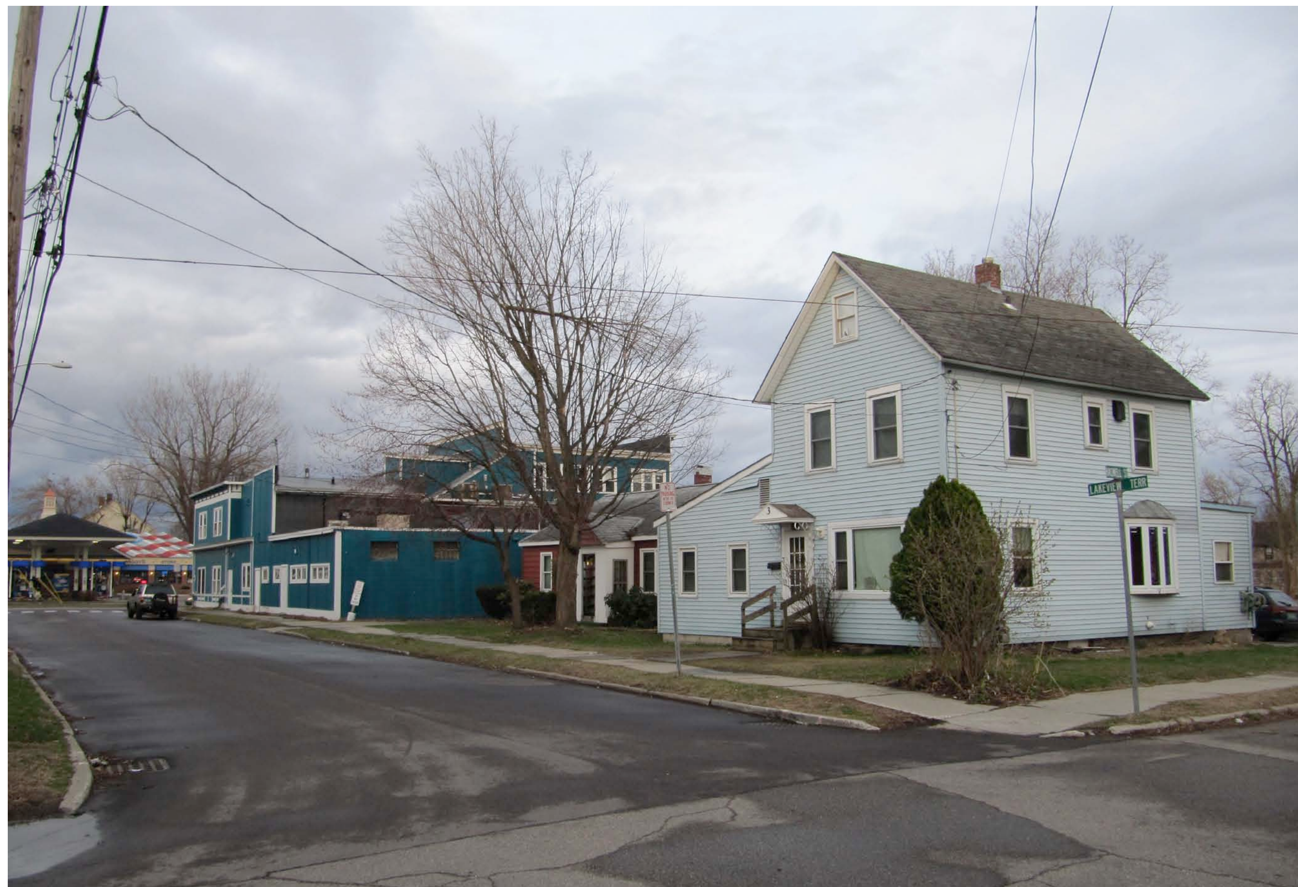
View looking east down Haswell Street
