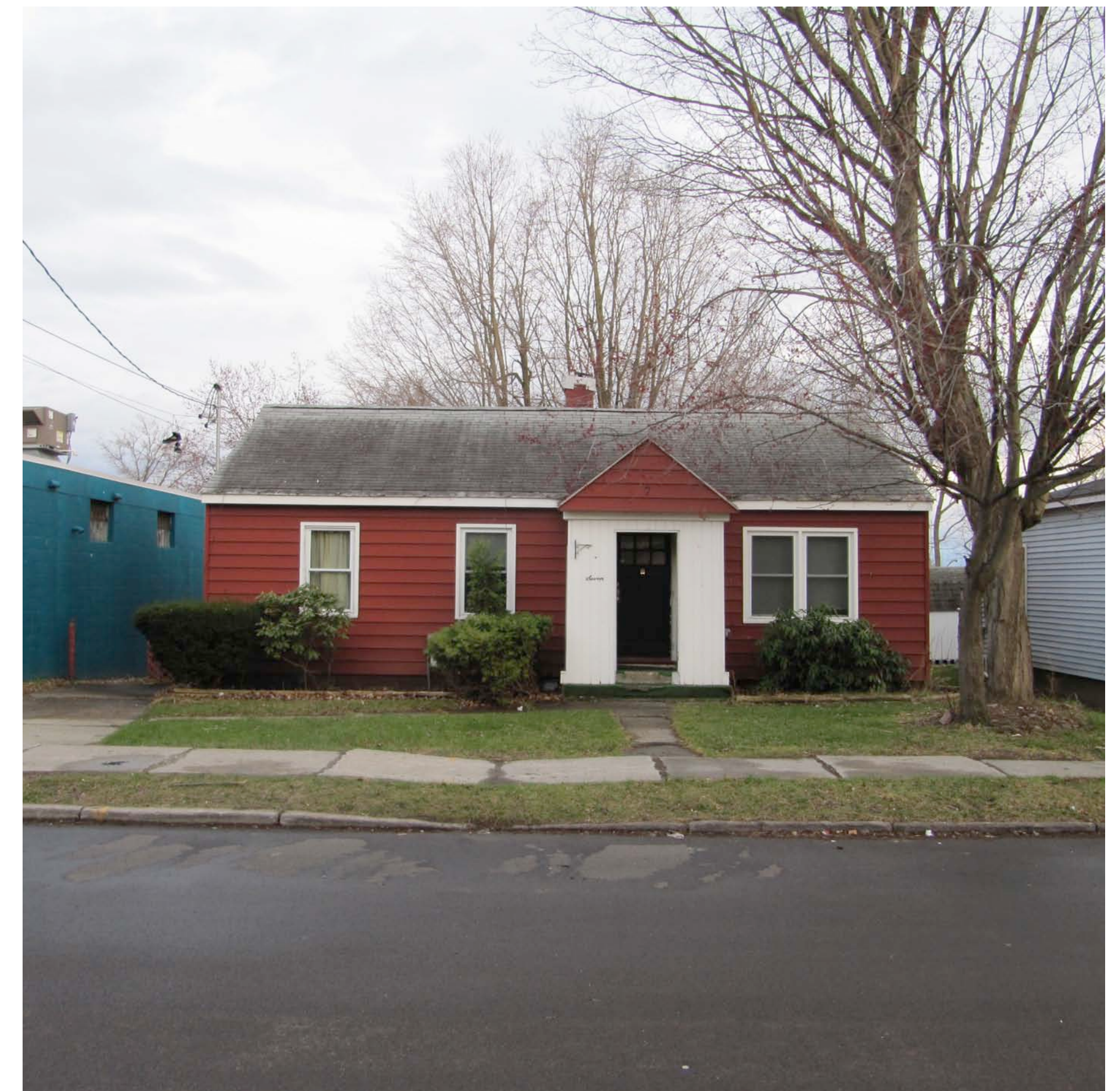
Adjacent property, to be removed
