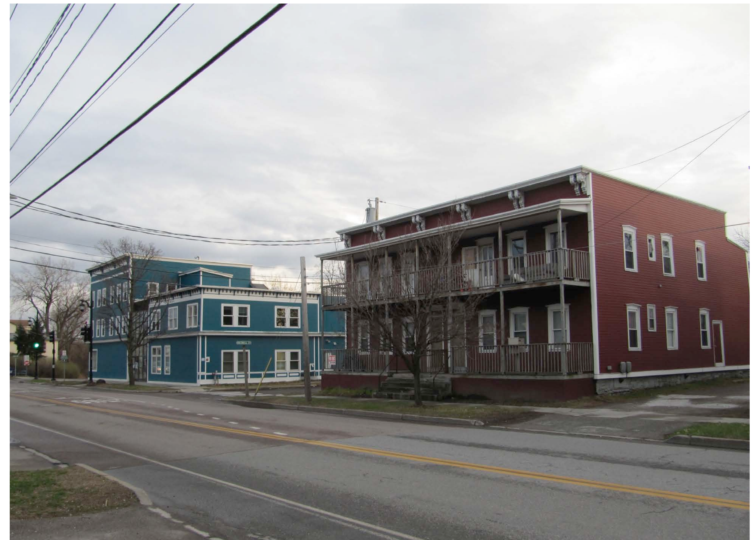
View looking southwest from North Avenue
