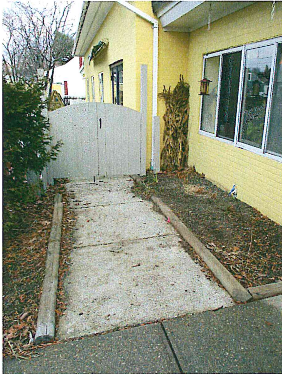
Main entrance looking north along existing building toward patio
