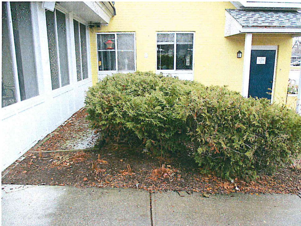
At existing main entrance looking south along existing building
