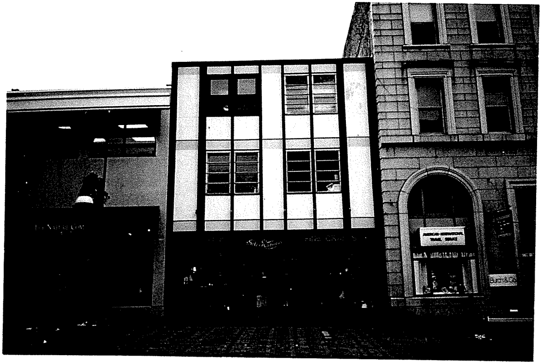
EXISTING STORE FRONT
