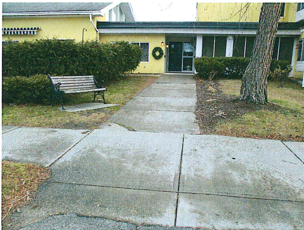
Existing curb cut at main walkway entrance looking east (location of new walkway)
