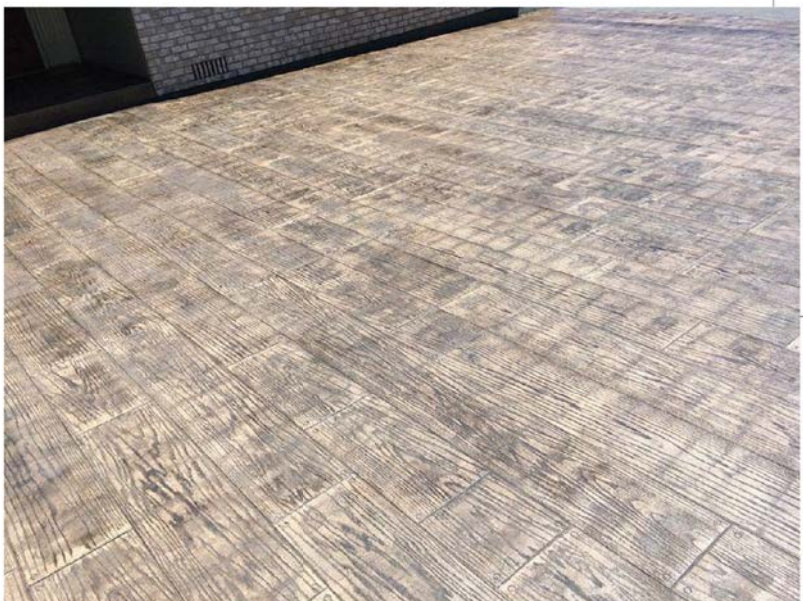
STAMPED BOARD FORM CONCRETE
