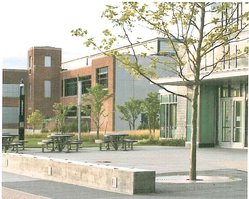
TREE IN GRATE and BOARDFORM CONCRETE SEATWALL Trees surrounding New Moran in round tree grates; curving boardform concrete seatwall separating stormwater area from plaza
