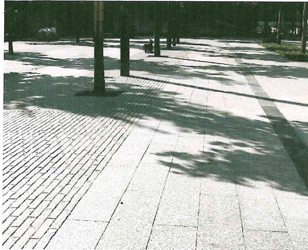
PAVING Banded concrete unit paving - promenade between Burlington Electric and New Moran (smaller pavers) and plaza (larger pavers)
