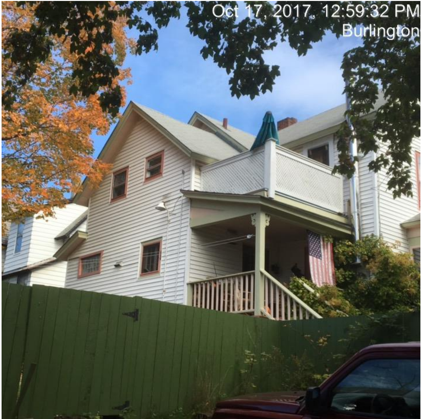
Deck and door were denied under ZP 17-1255CA on September 6. This fence style, solid fence, has replaced a picket fence.
