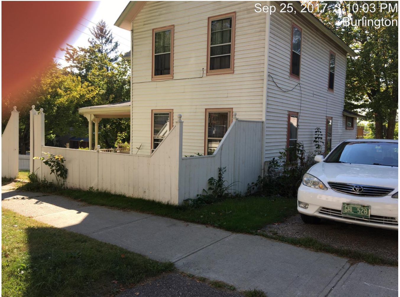
Front yard fence higher does not comply with permit.
