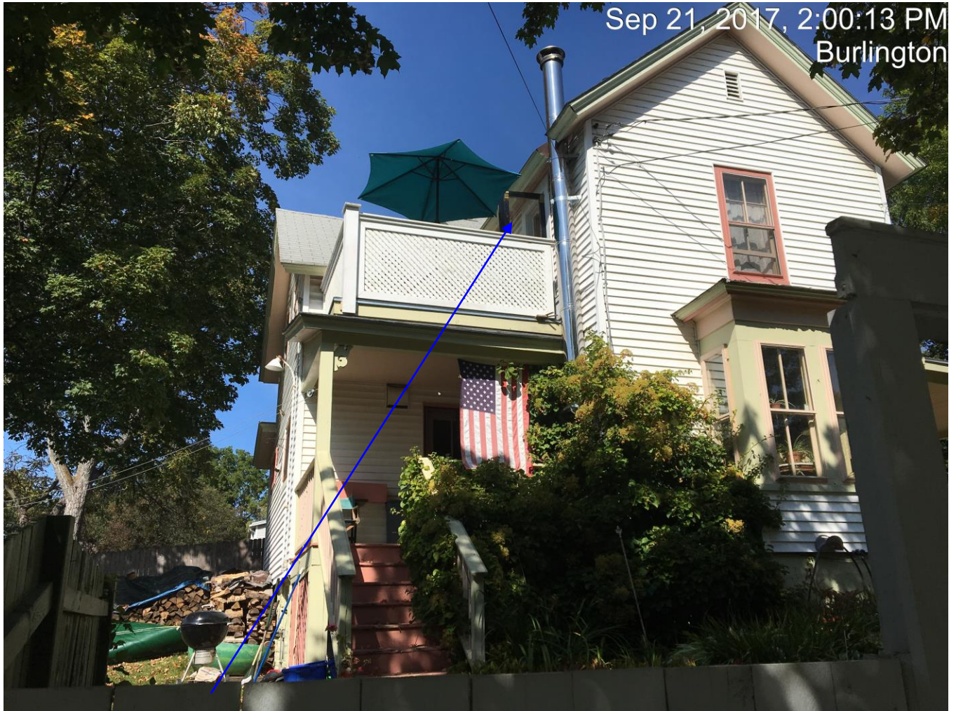
Roof top deck with access door on southwest corner of house were denied zoning approval on September 6, 2017.
