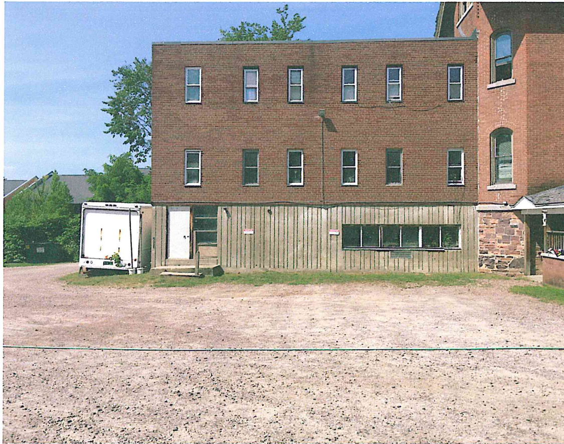
Current Rear of Building – South Elevation
