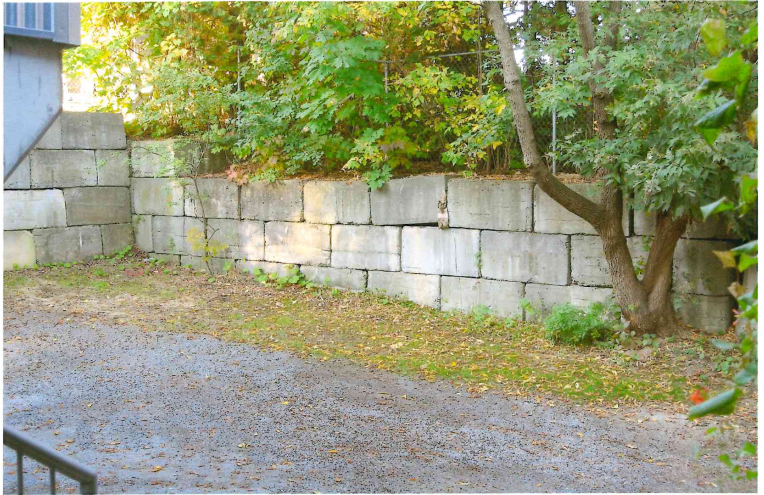
General view of south wall and west wall
