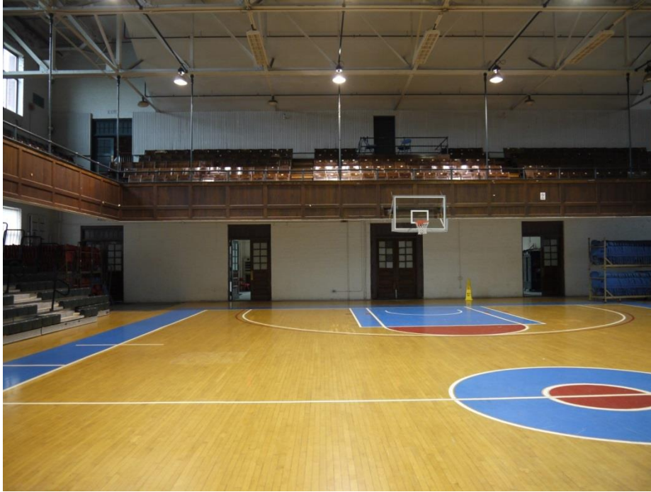
Auditorium – Looking West toward Lobby
