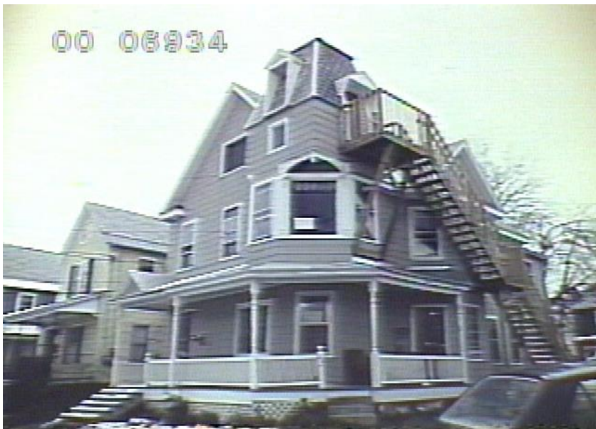
1984-85 Assessor Revaluation photograph Stairs are new build
