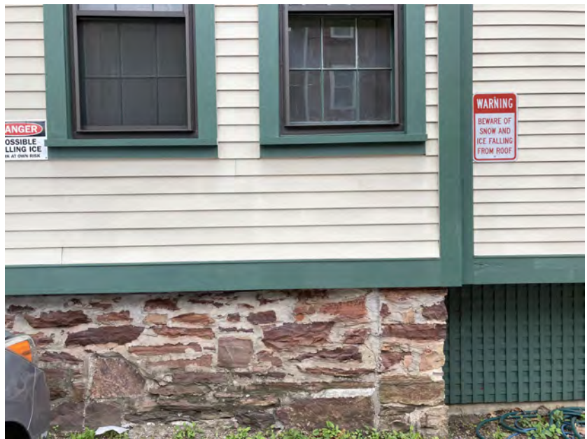
EXISTING STONE FOUNDATION
