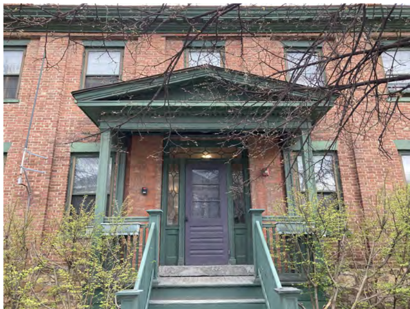
FRONT OF EXISTING BUILDING, SOUTH SIDE
