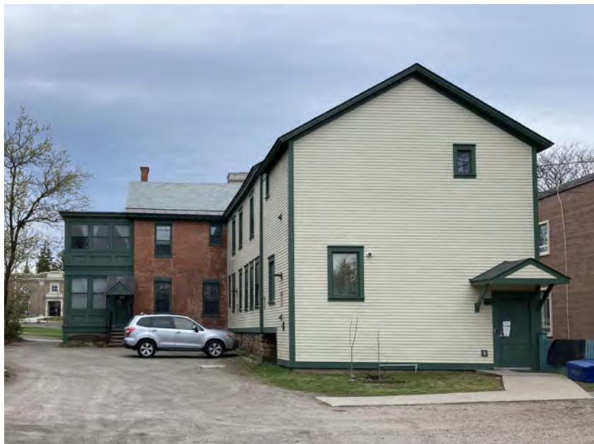
REAR OF EXISTING BUILDING
