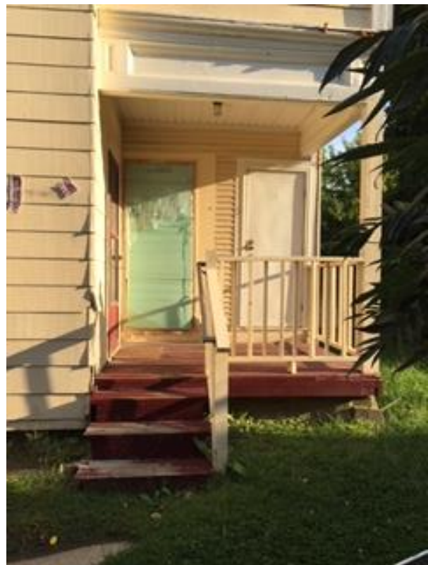
First floor south/east entry; entry door appears to have been relocated, one door sealed off.
