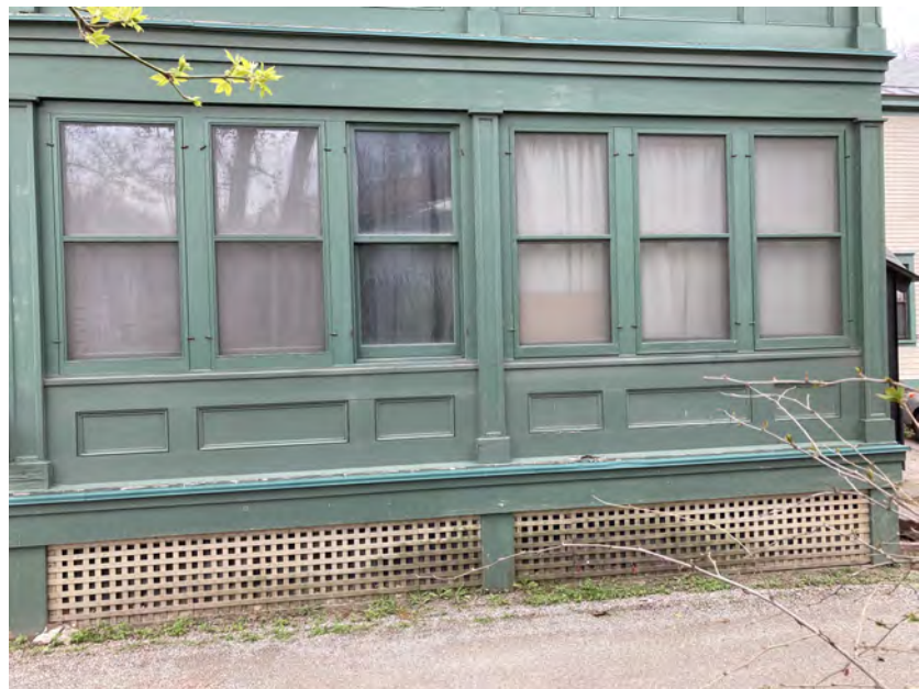
EXISTING STONE FOUNDATION
