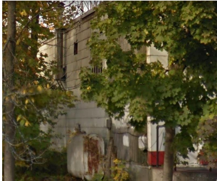
West elevation (rear), 2014 street view Siding appears to be asbestos shingle
