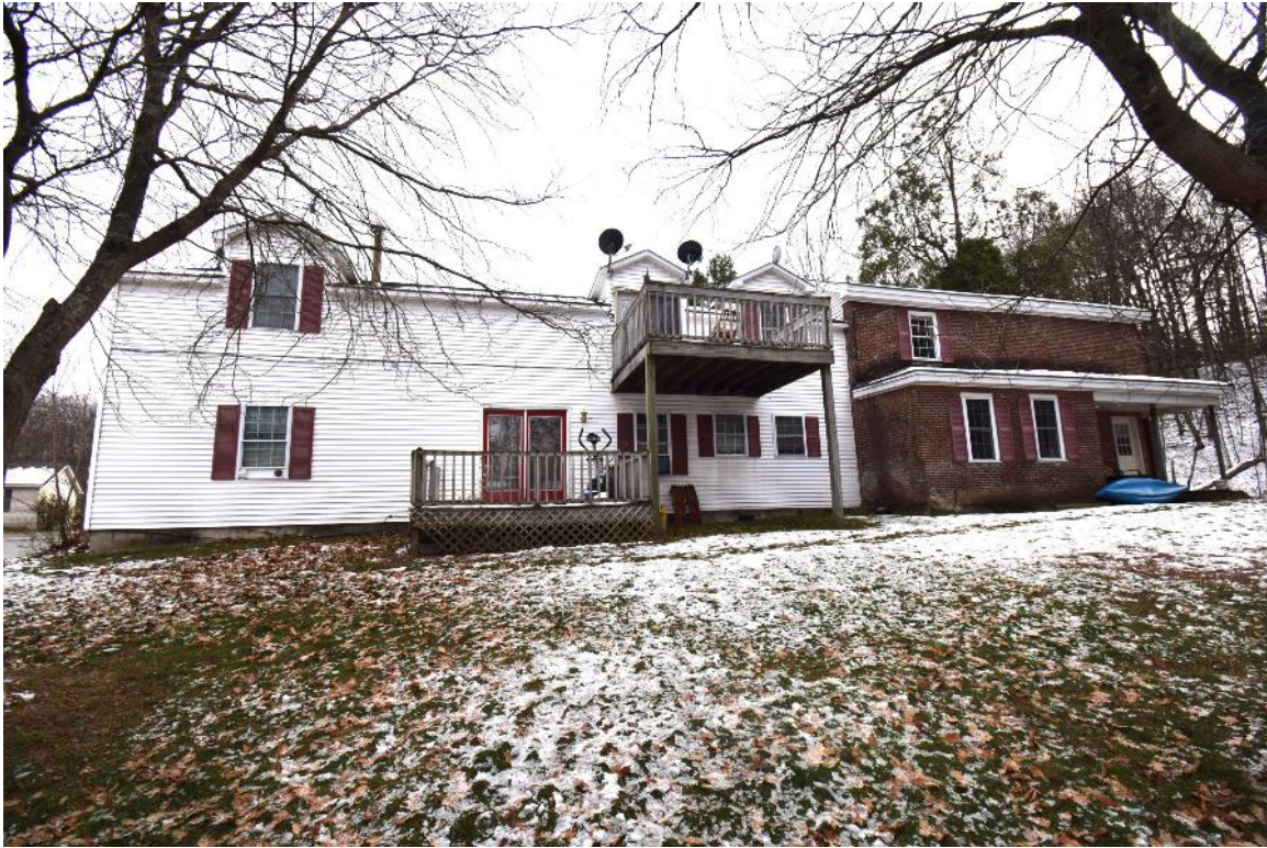
Figure 16: Looking east, view shows main block and addition west elevations
