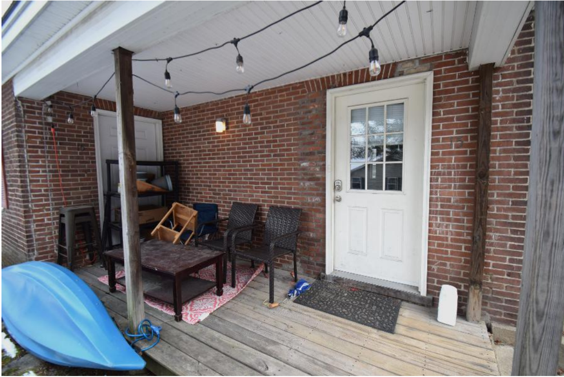
Figure 22: Looking northeast in main block west elevation entrance porch
