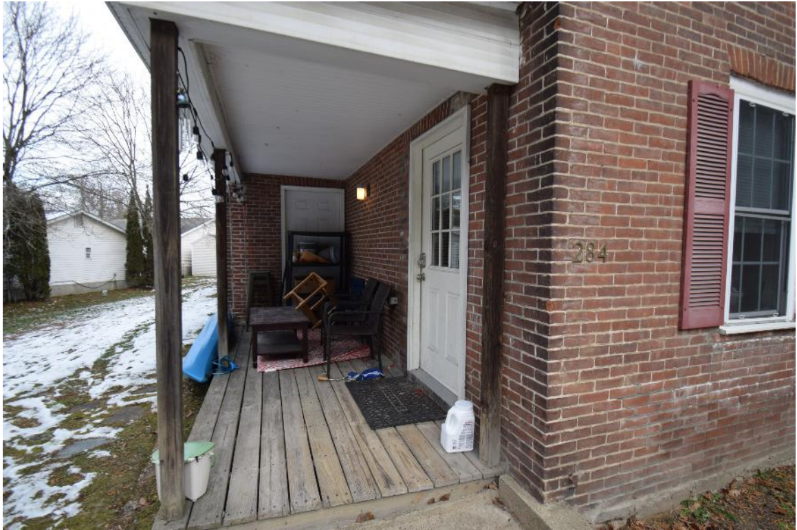
Figure 32: Looking north, view shows altered, half-enclosed porch with trim clad in vinyl
