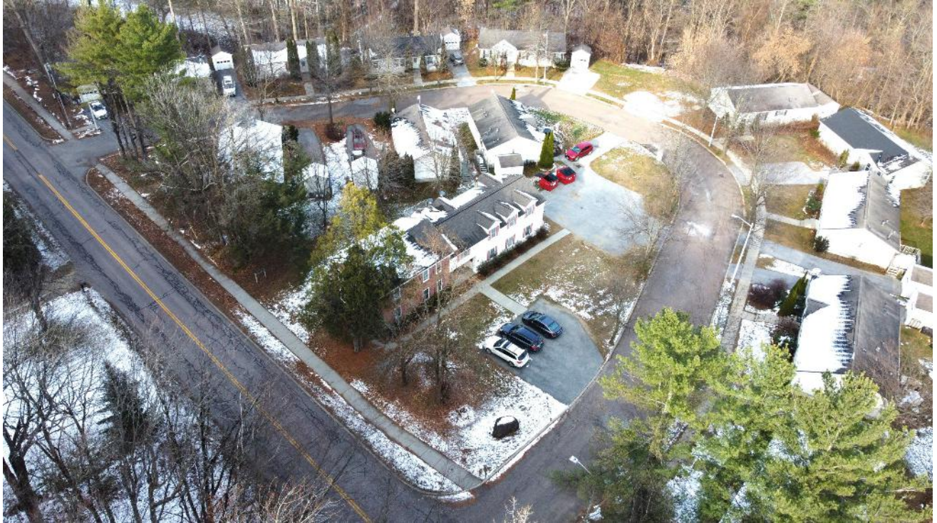
Figure 08: Looking northwest, aerial image shows 284 Grove Street and surrounding modular home development
