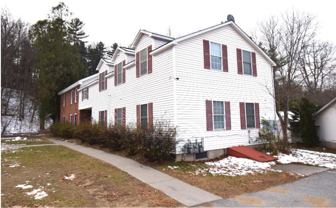
Figure 18: Looking southwest, view shows rear addition
