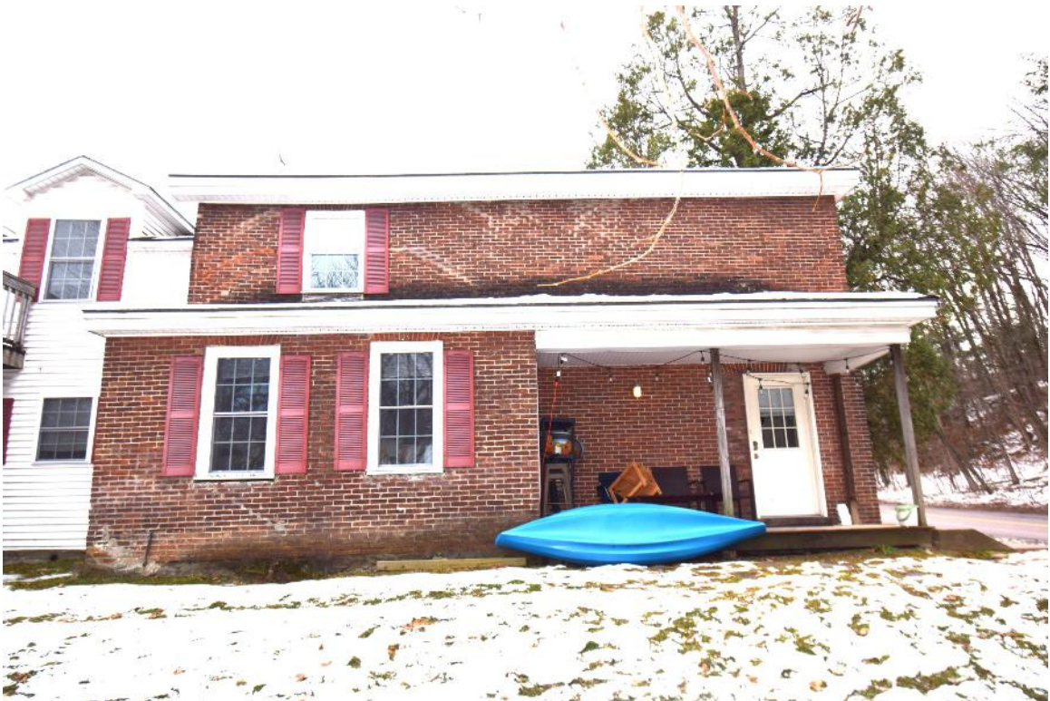
Figure 15: Looking east, view shows main block west elevation, formerly an open porch
