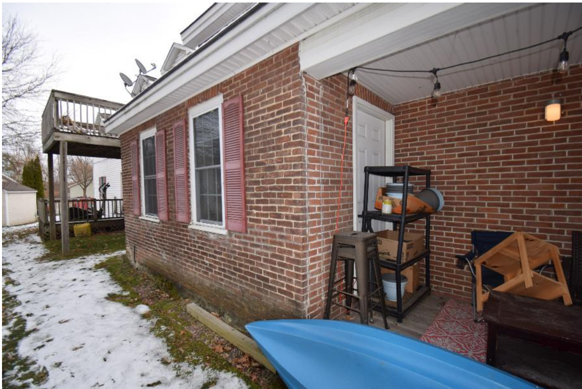
Figure 23: Looking northeast in main block west elevation entrance porch
