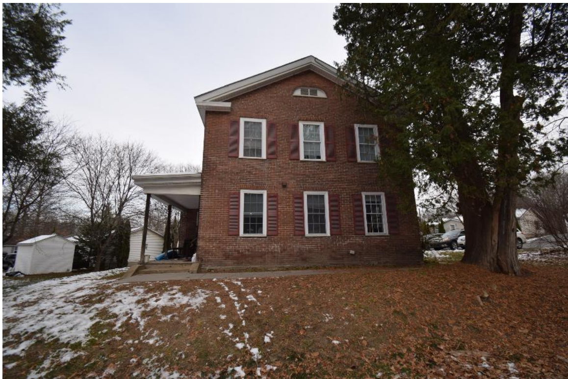
Figure 13: Looking south, view shows 284 Grove Street facade
