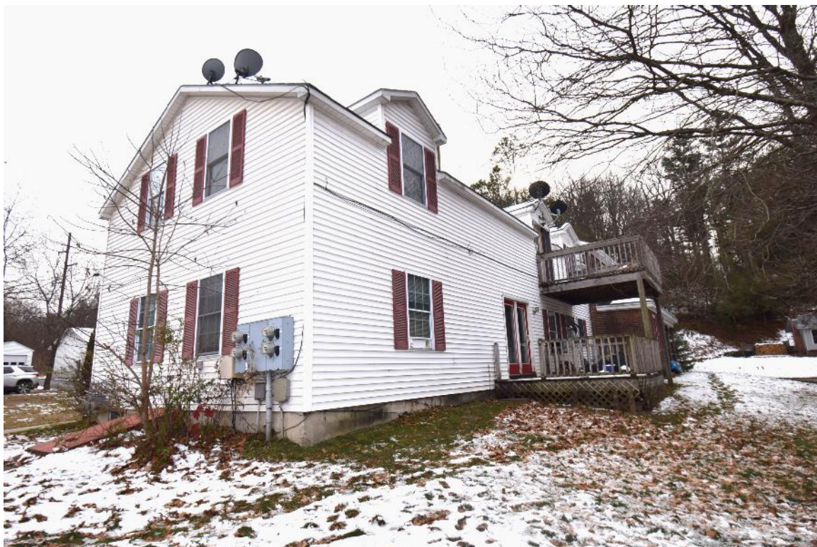
Figure 17: Looking southeast, view shows modern rear addition
