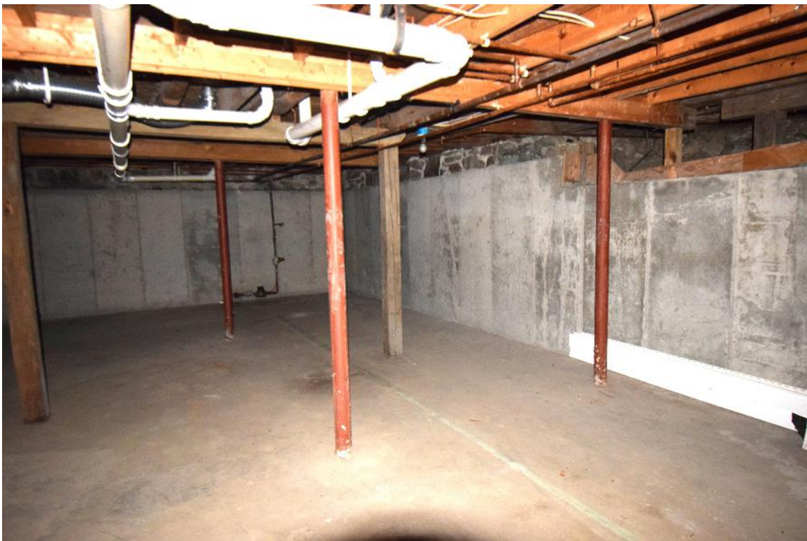
Photo XX: Looking south in main block basement, the stone foundation has been covered with a full height concrete wall
