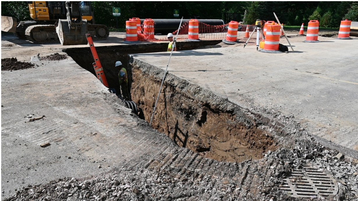
Figure 26. View of the location of the wooden plank lined subsurface feature, looking southwest (2021) (see the middle of trench directly above the ladder's shadow).
