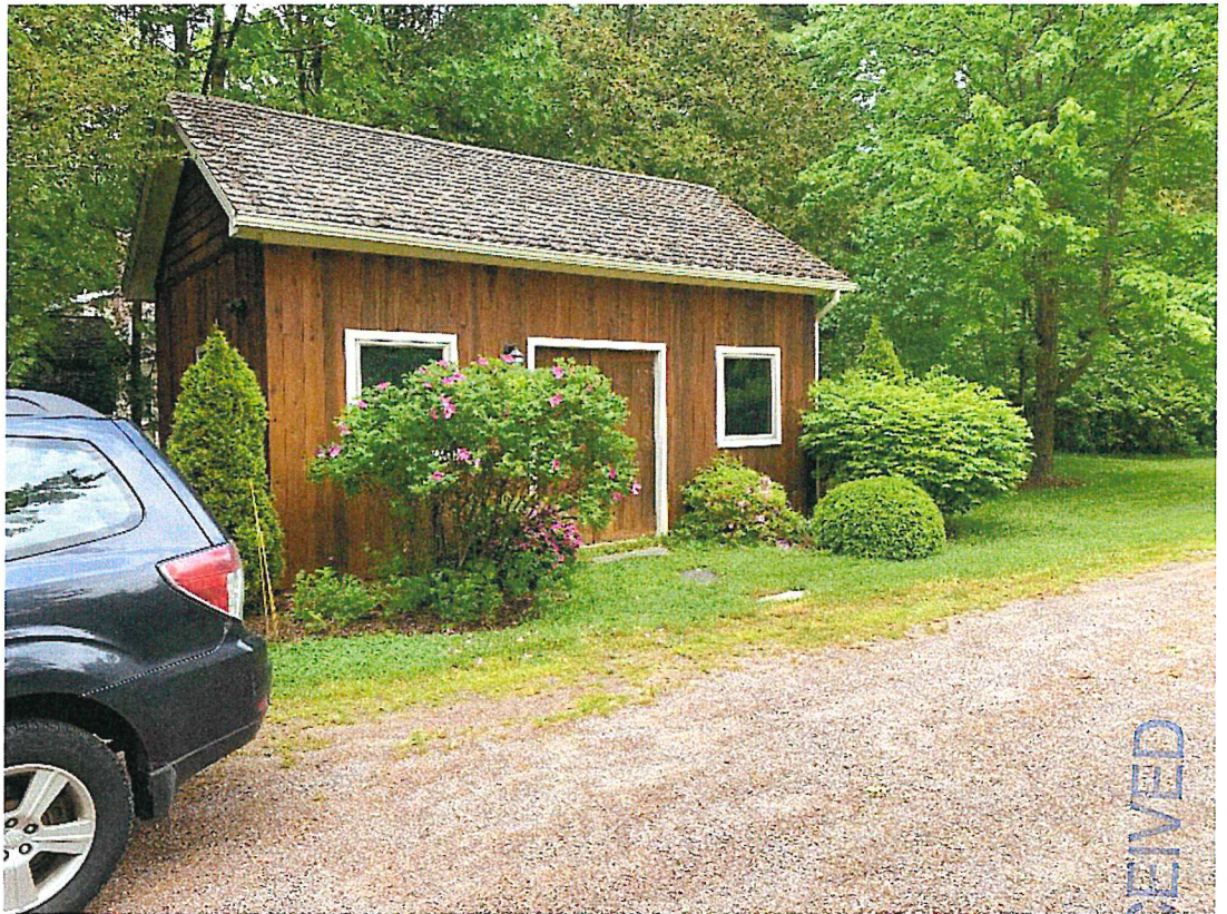
5b Looking east from the project driveway at the existing shed
