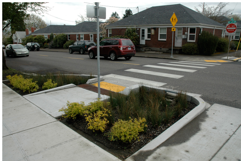
Stormwater Curb Extension in Portland, OR
