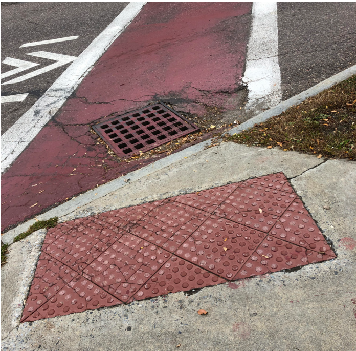
A stormwater inlet interrupts the crosswalk. Crosswalk markings do not meet current best practices for high visibility, and the detectable edge is cracked and awkwardly placed.
