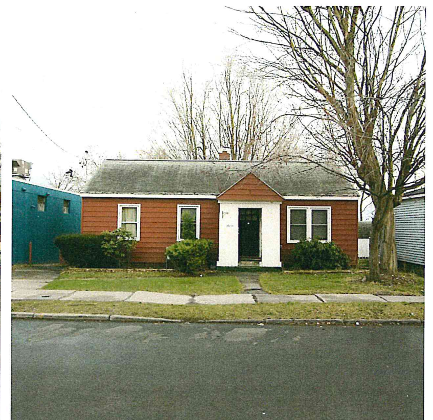
Adjacent property, to be removed
