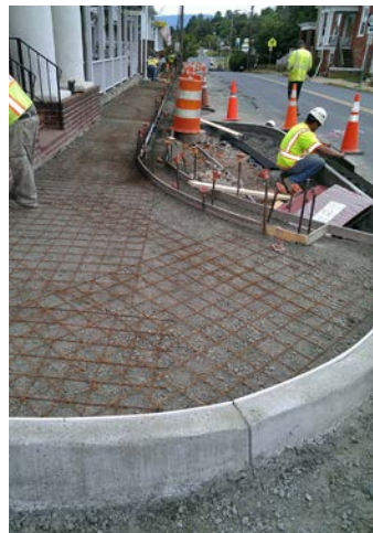
Construction of a curb extension, or "bumpout"
