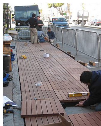
Installation of parklet platform in the Parking Lane
