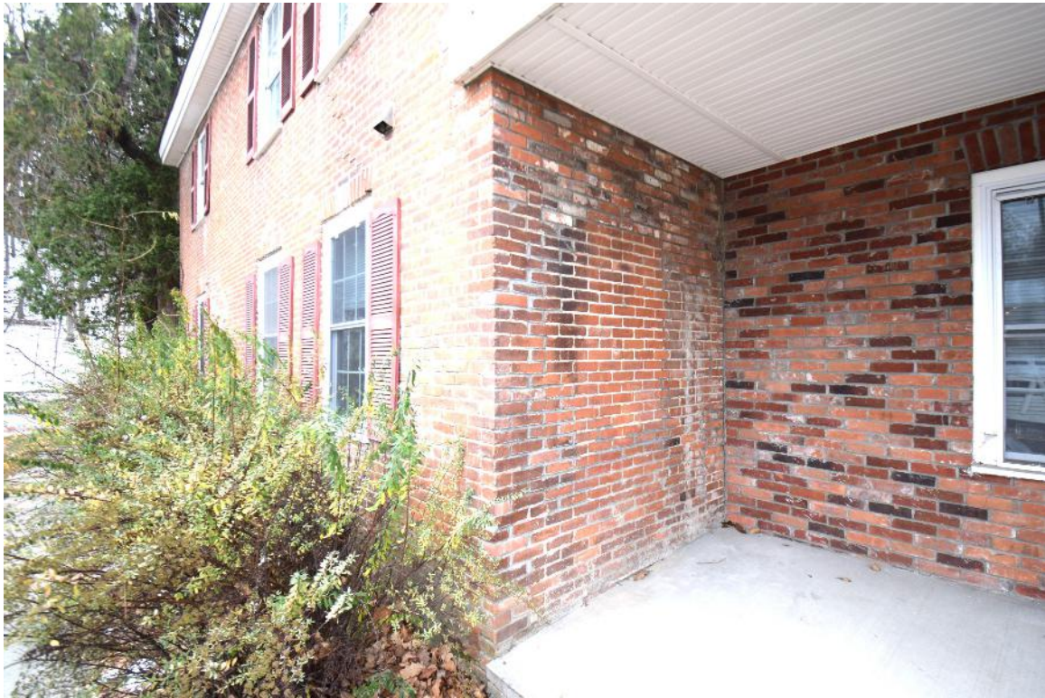
Figure 30: View shows what appears to be a closed in window, rebricking of the wall at right, and new door and window
