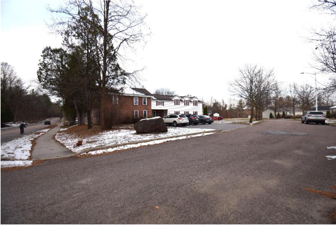
Figure 10: Looking west along Grove Street with #284 in frame center
