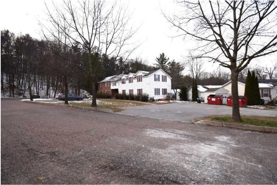
Figure 12: Looking northwest from the development loop road, view shows large addition attached to 284 Grove Street
