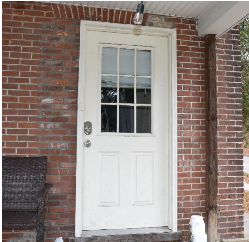
Figure 24: Looking east at main block west elevation fiberglass entrance door, note relocation of the door to the south
