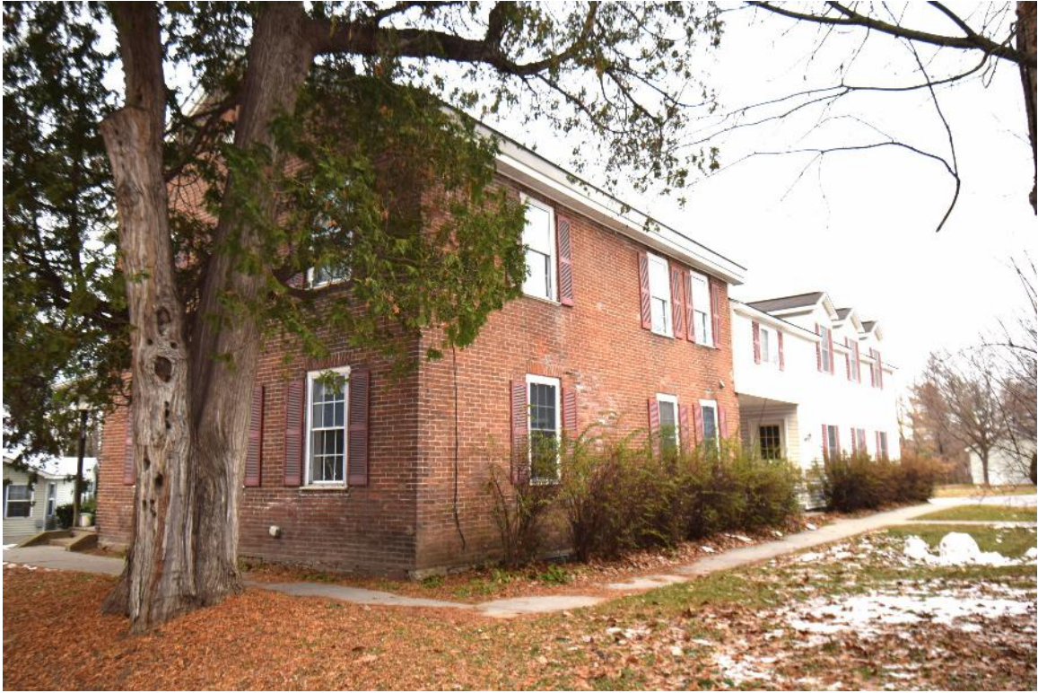
Figure 20: Looking northwest, view shows main block façade and east elevation
