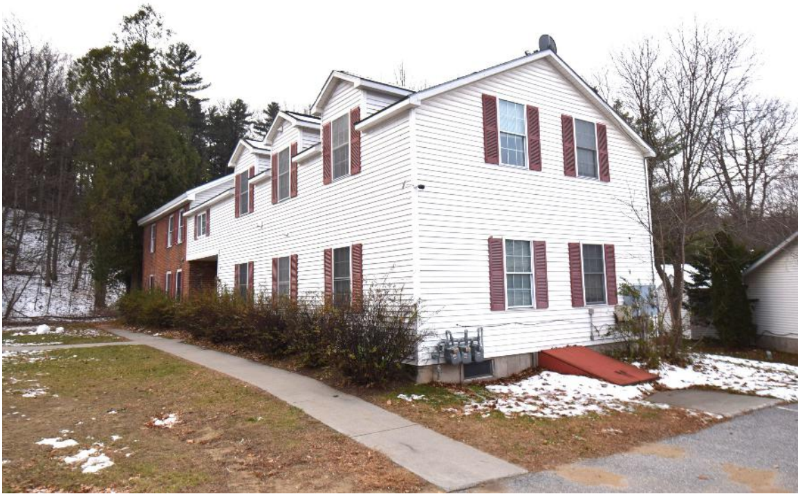
Figure 18: Looking southwest, view shows rear addition
