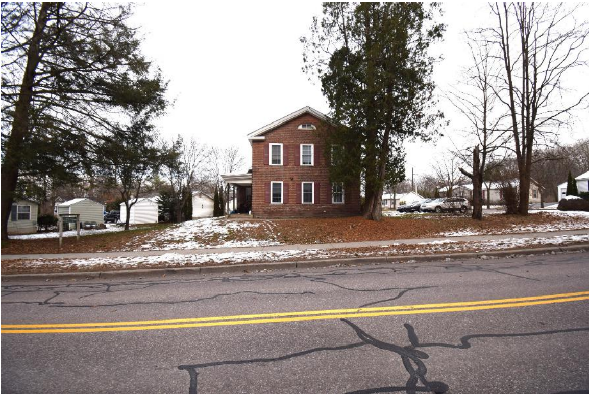
Figure 11: Looking north from the south side of Grove Street
