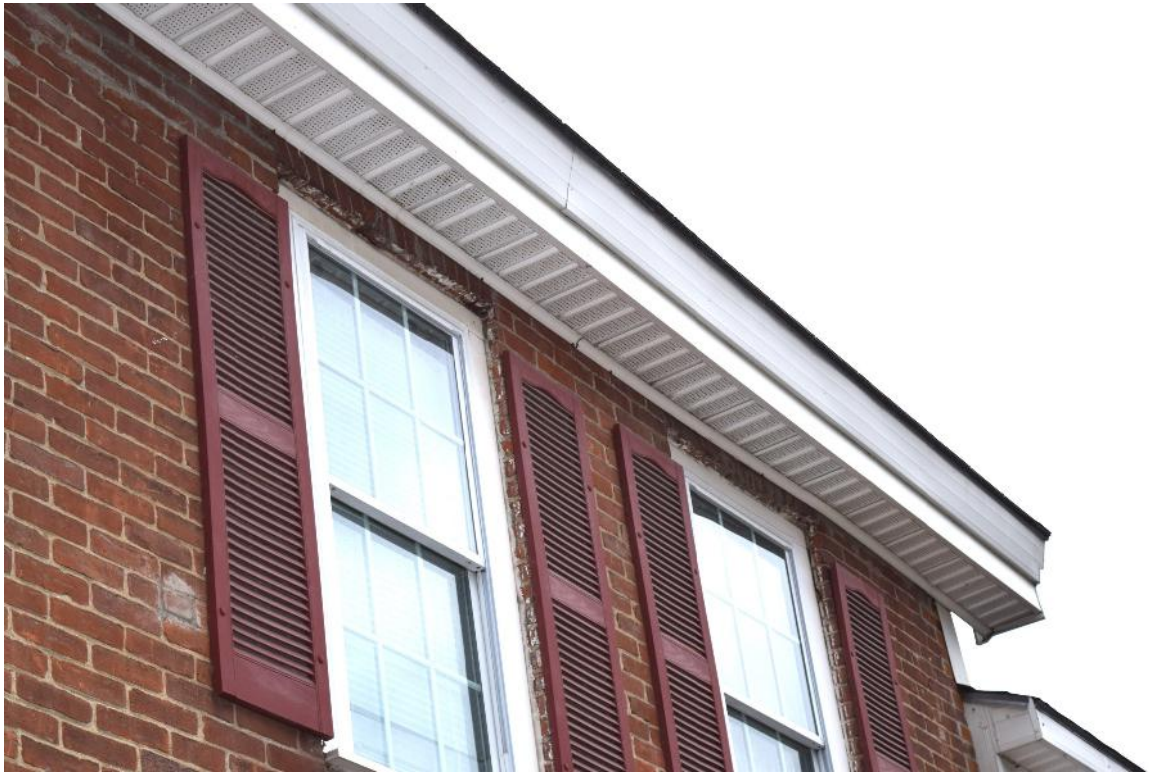
Figure 34: View shows typical treatment of trim, uniformly clad in vinyl
