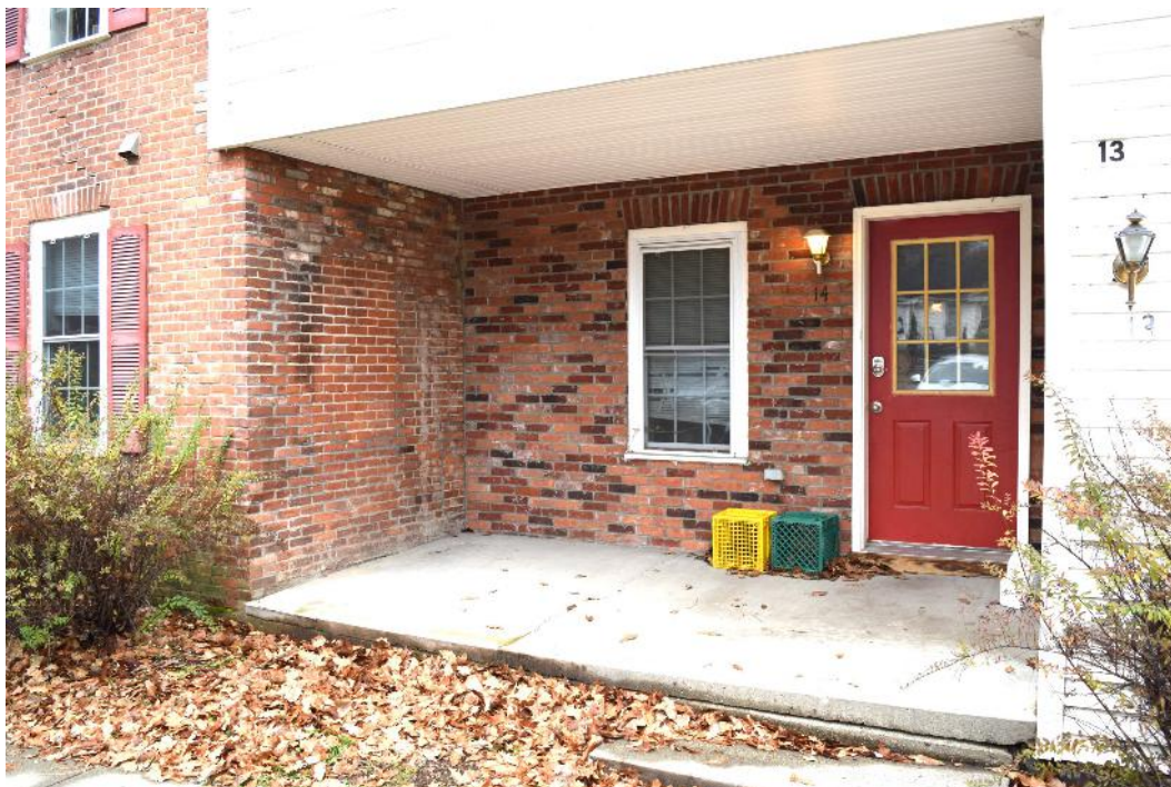
Figure 21: Looking west, view shows recessed entrance at south end of addition. This is on the footprint of an early addition but has been rebricked. See photo # XX for the brick chimney previously at this location.
