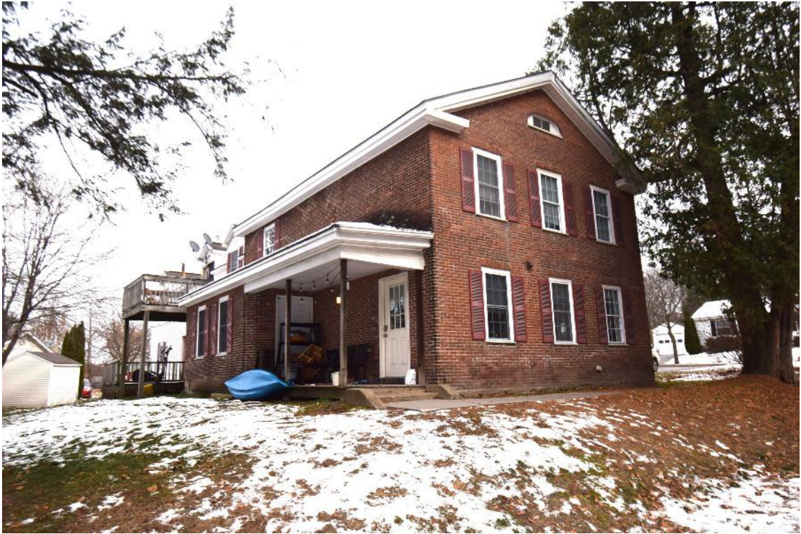
Figure 14: Looking northeast, view shows west elevation (left) and façade (right).
