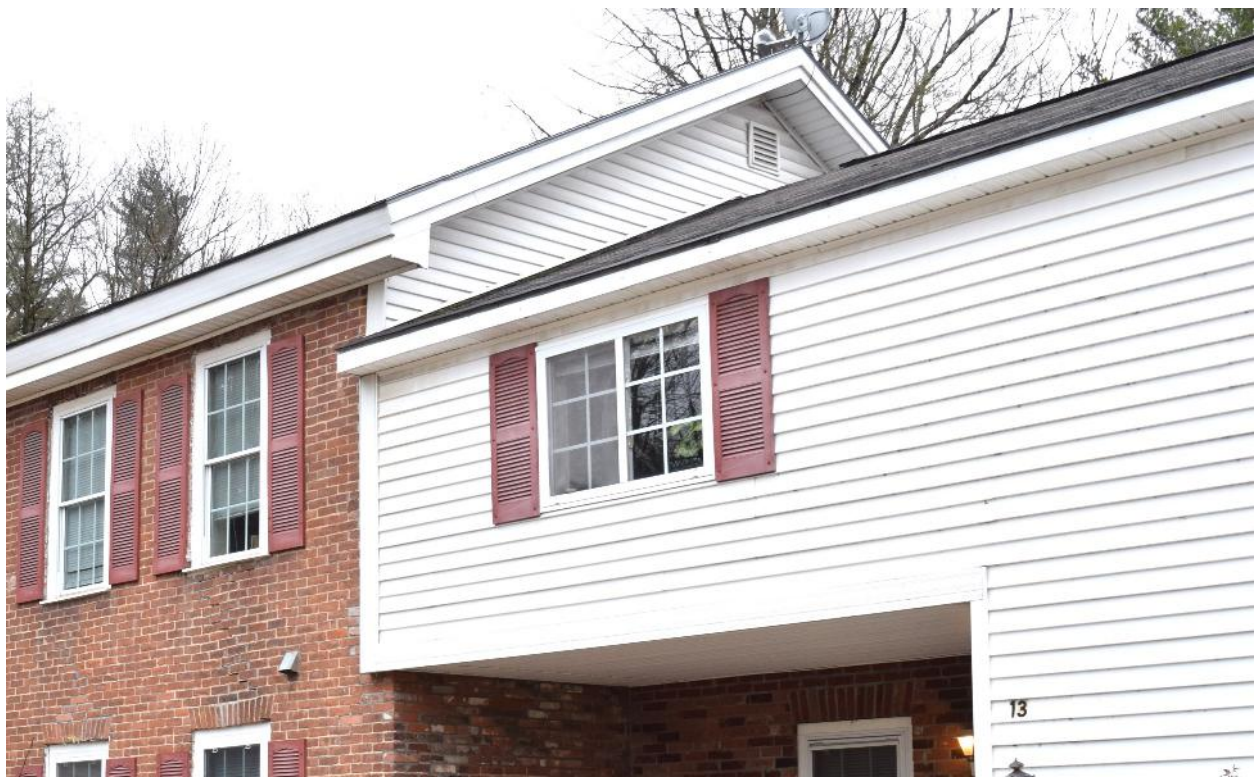
Figure 33: Looking southwest, view shows vinyl clad gable on main block where the plywood covered addition previously attached to the main block
