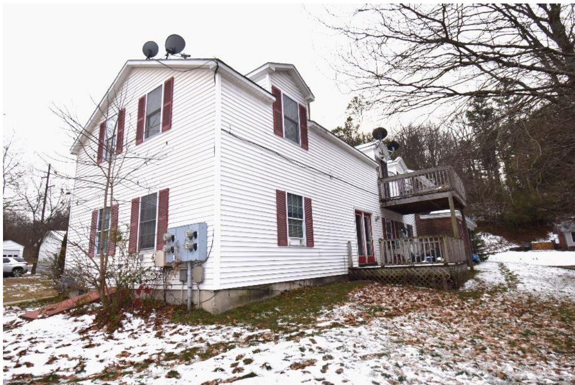
Figure 17: Looking southeast, view shows modern rear addition
