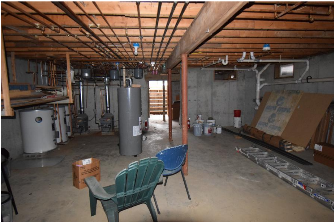
Photo XX: Looking north in the addition basement which has a poured concrete foundation
