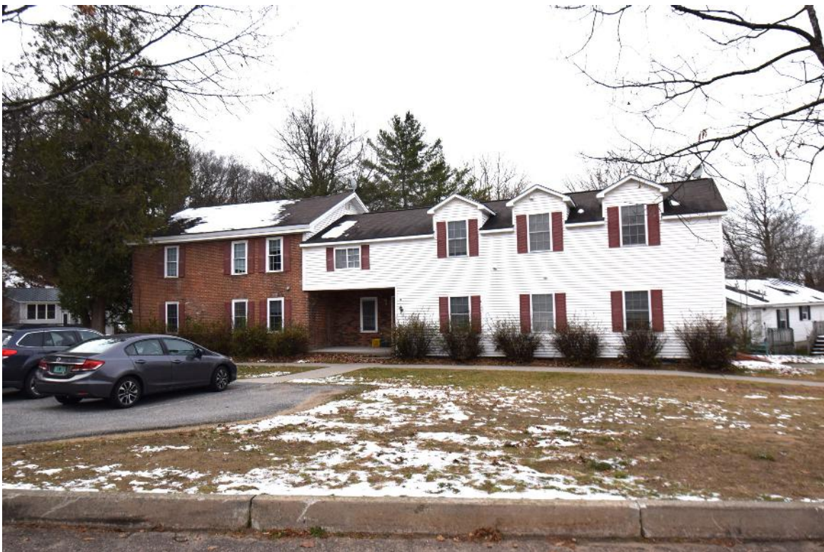
Figure 19: Looking west, view shows east elevation of main block and addition
