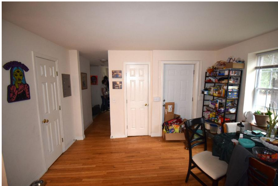
Figure 39: Looking south in first floor interior which has been reconfigured, sheetrocked, and remodeled with new floors, fiberglass doors, and trim.
