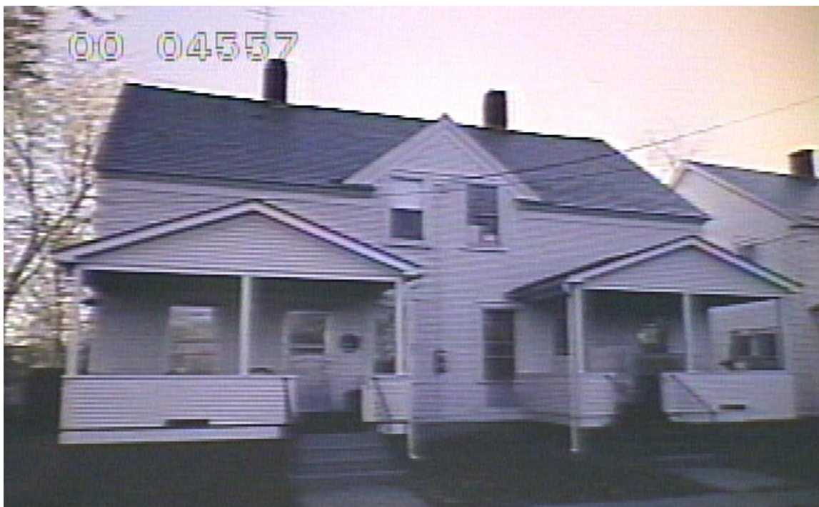
1984-85 Assessor Revaluation photograph Note window casing details
