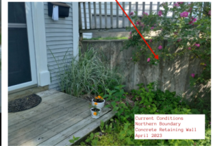
Existing Concrete Retaining Wall - July 2011
