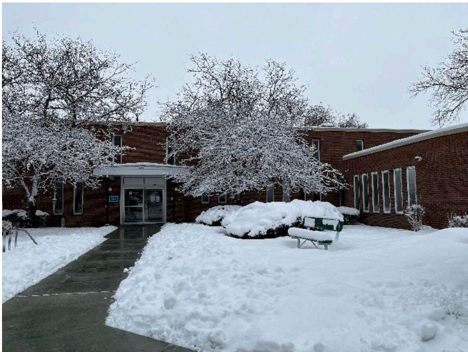
FLYNN AVENUE ENTRANCE
