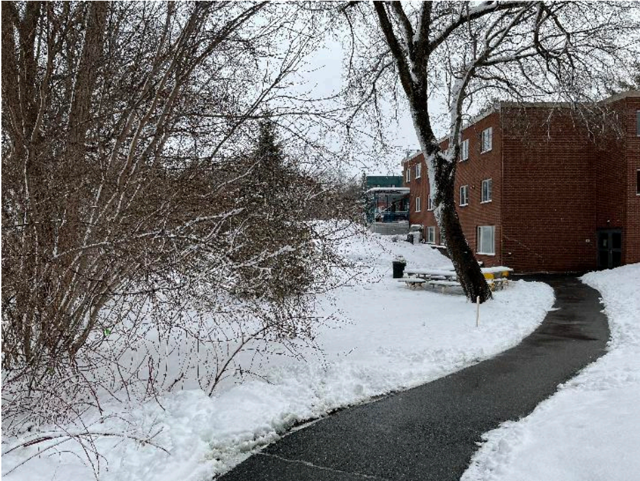
NORTH SIDE OF BUILDING
