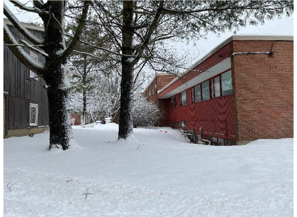
VIEW FROM PINE STREET
