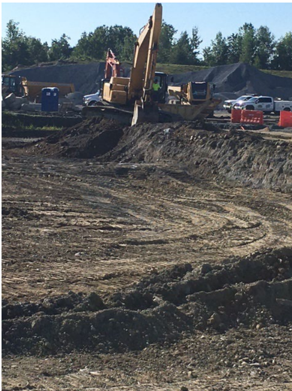
Apron Excavation for Subgrade Materials Placement
