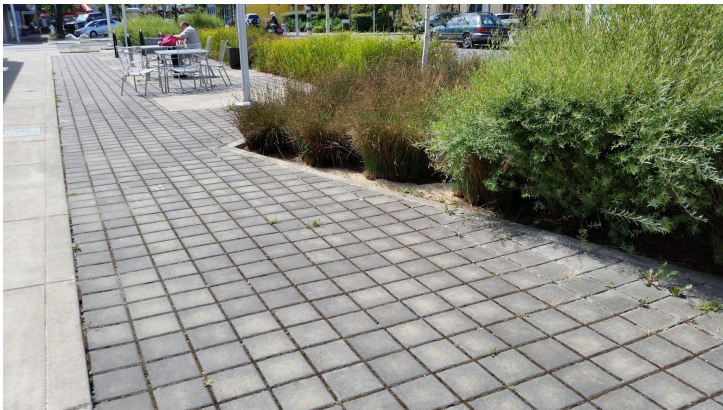
Patio Flooring Permeable Concrete Pavers
