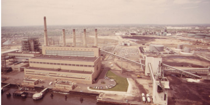
Figure 3.8: The Searles Generating Station in New Jersey. Source: Ike Voss, Environmental Protection Agency.
