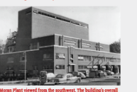
Moran Plant viewed from the southeast. The building's overall form reflected its historic industrial use, with the highest portion housing the hoppers that fed coal to the boilers. Source: Burlington Electric Department
