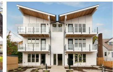
North Emerson Street - Portland, OR
