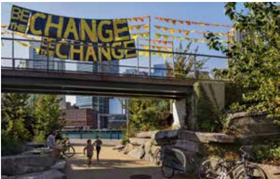
Pedestrian Bridges Connect Park Levels
