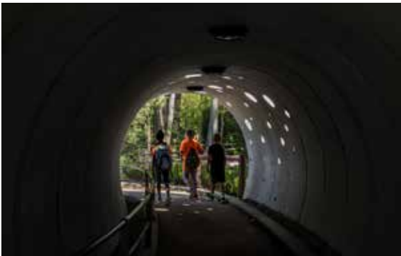
Pedestrian Tunnels and Bridges
