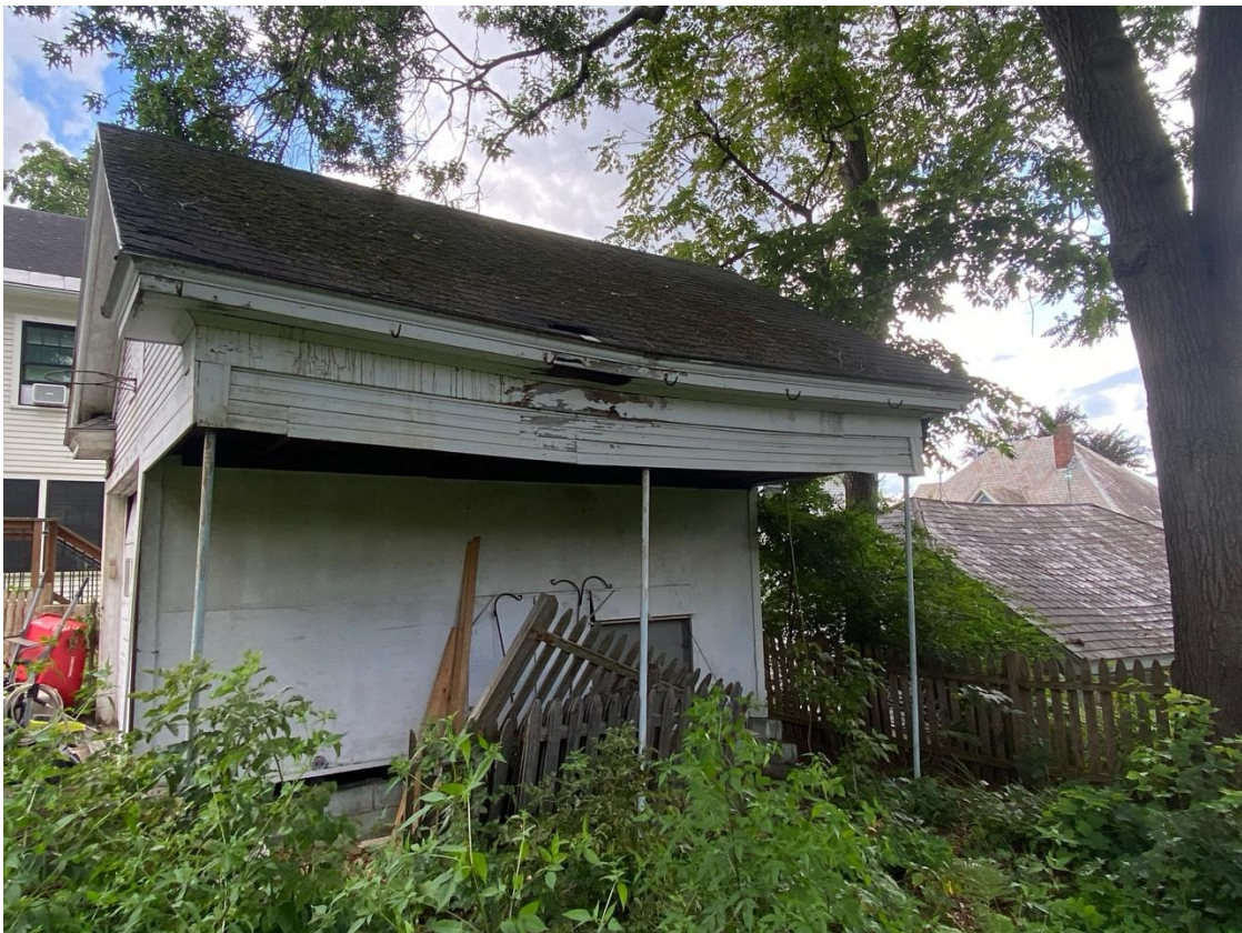
-Top Plate is bowed and sagging
