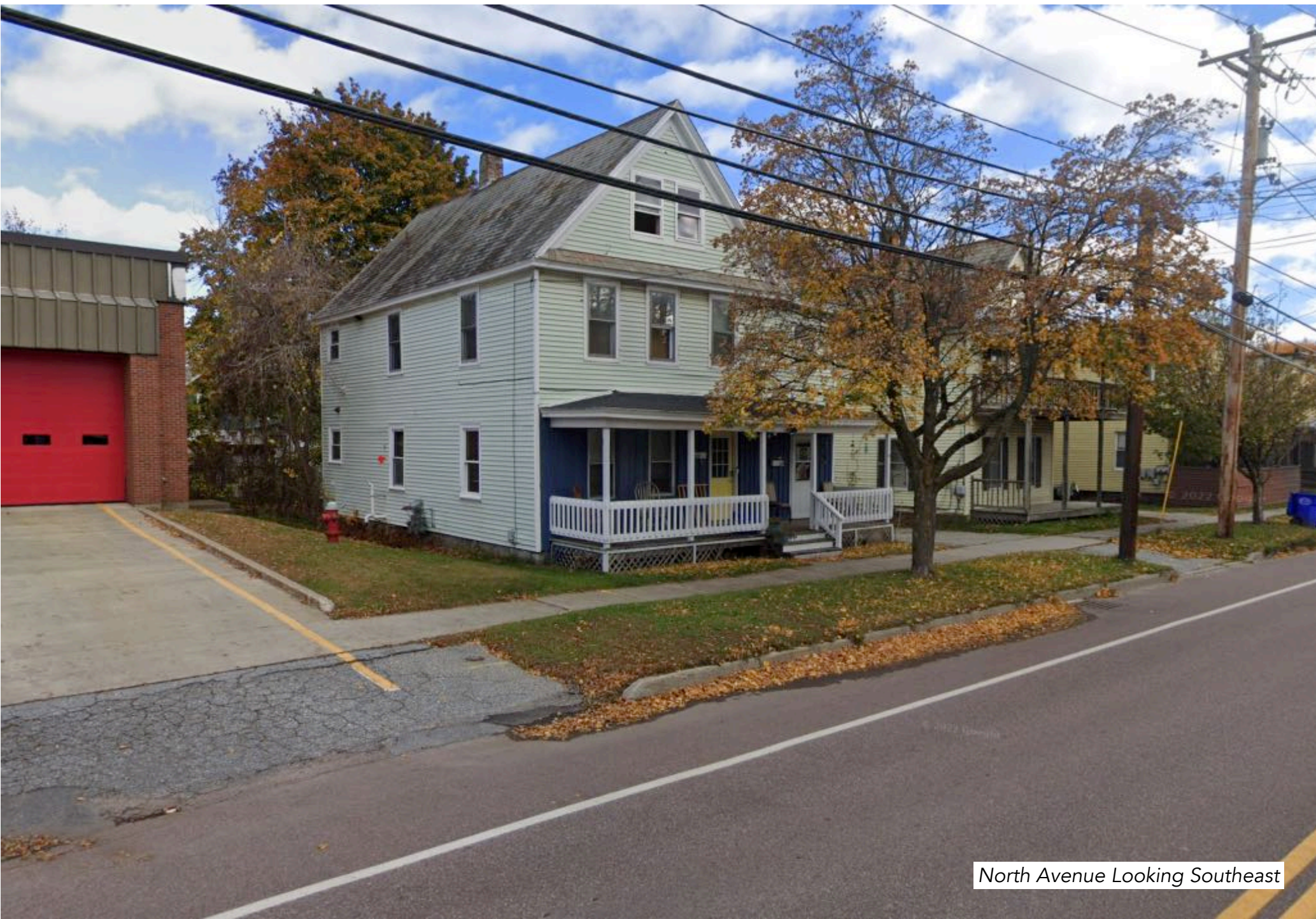
3 Existing Conditions Photograph Scale: None
