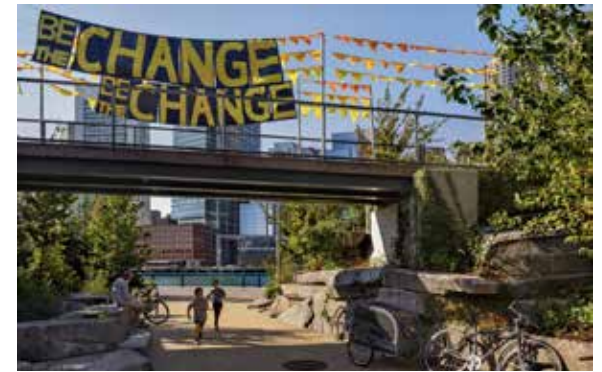
Pedestrian Bridges Connect Park Levels
