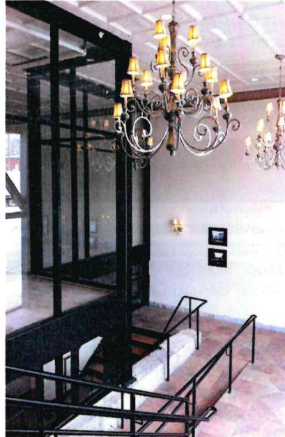
Blanchard Block, West Lobby. Provides ADA access by removing part of first floor to create tall lobby space off west parking entrance to reach new elevator.
